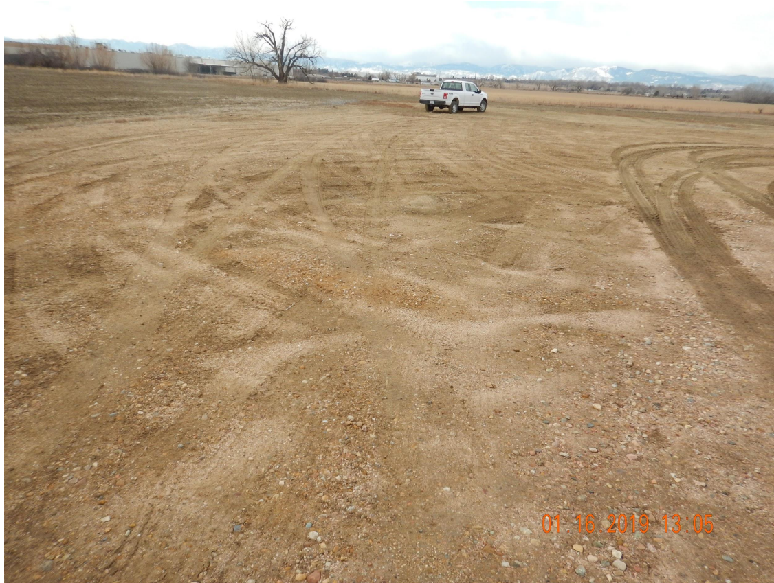
Photo 1. Photo taken from the southwestern well pad, facing West. Operator has failed to perform interim reclamation to reduce disturbance areas only needed for production operations. Also, there was stormwater erosion observed along the western and southwestern location discharging off location.
