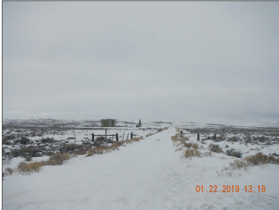
Photo 1. Overview of access road from county road. No winter maintenance apparent.
