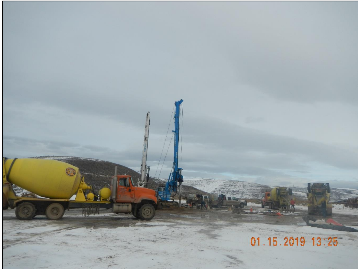
Ready mix cement trucks for conductors
