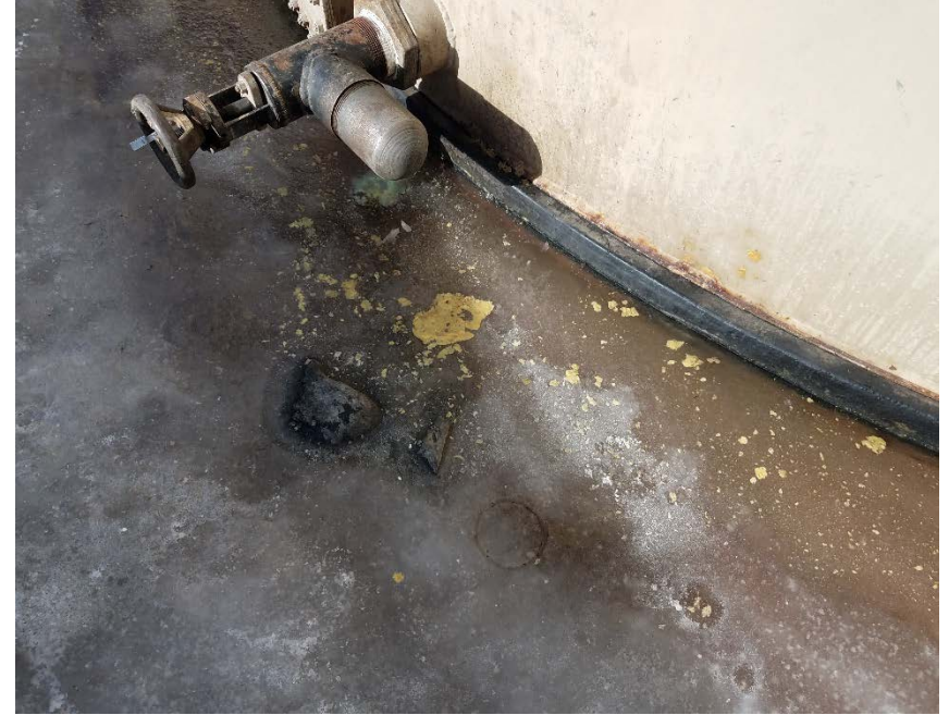
Location Photo #4, Condensate in battery containment.
