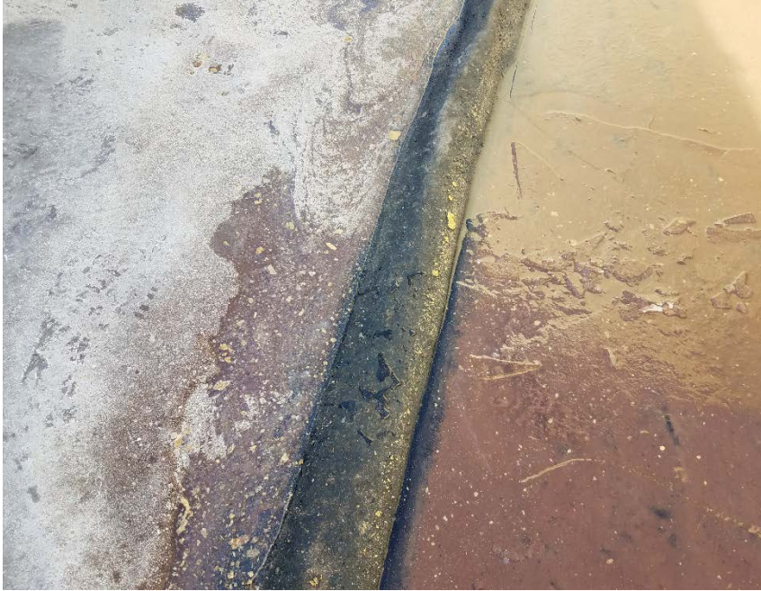
Location Photo #5, Condensate in battery containment.
