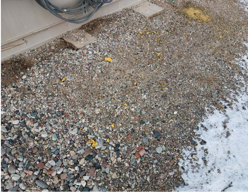
Location Photo #7, Condensate on ground by separator.
