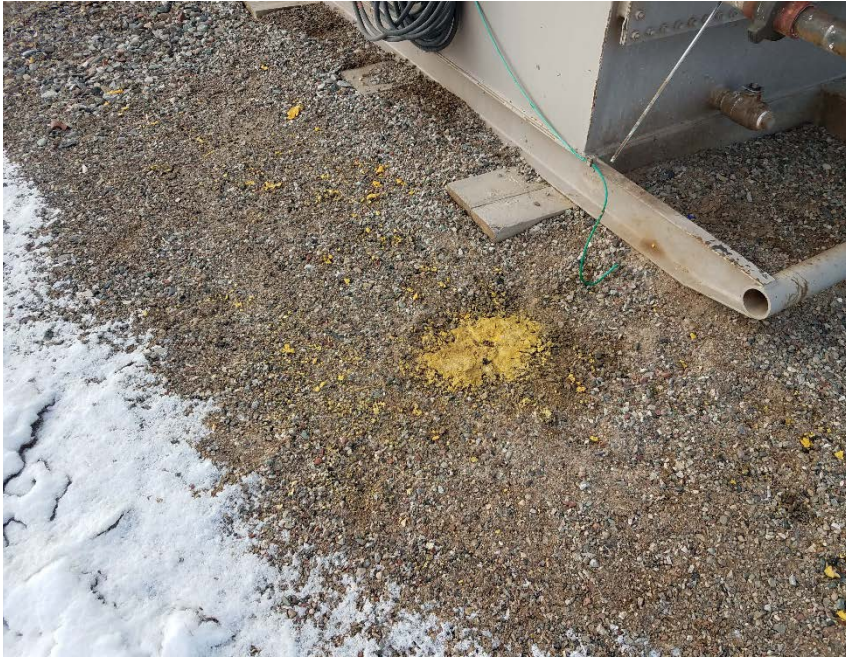
Location Photo #5, Condensate on ground next to separator.
