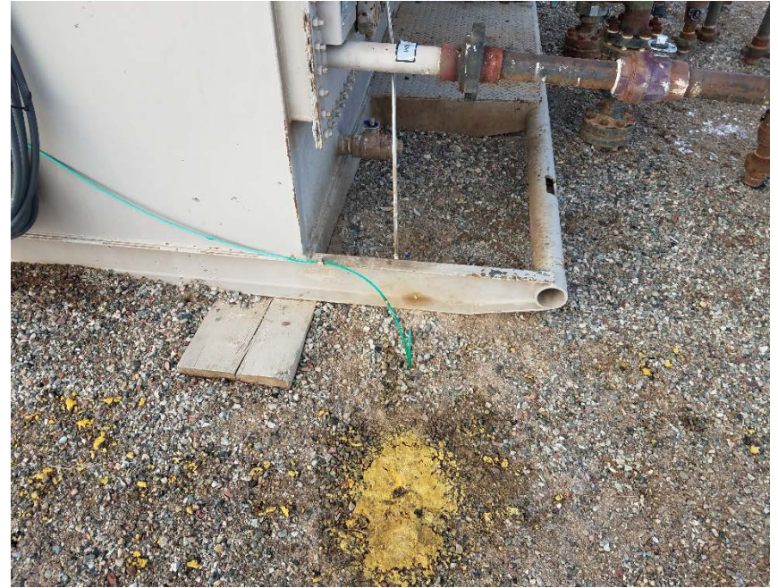
Location Photo #6, Condensate on ground next to separator.
