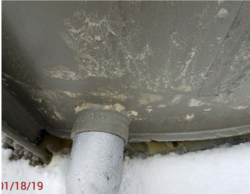
Location Photo #9, Condensate around base of tanks.
