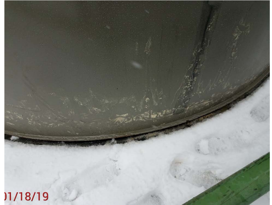
Location Photo #8, Condensate around base of tanks.
