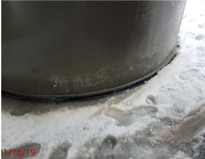
Location Photo #5, Condensate around base of tanks.
