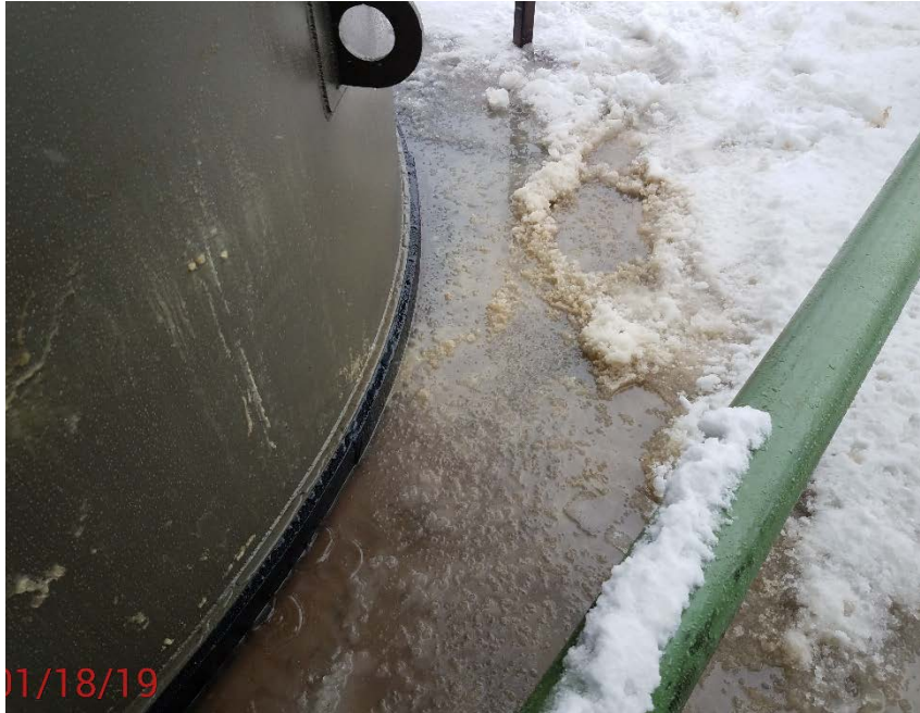
Location Photo #7, Condensate around base of tanks.
