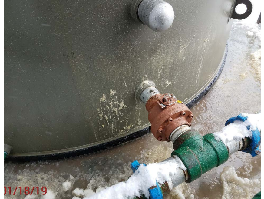
Location Photo #6, Condensate around base of tanks.
