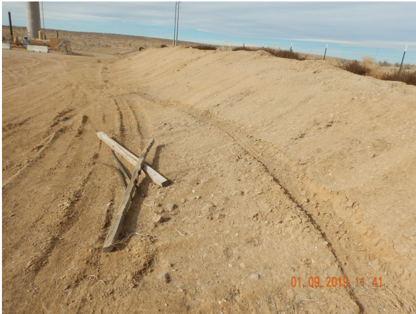
Photo 9. Photo taken from the northern location, facing West. Tackifier was observed on the cut slope but appears to be in need of maintenance. Also, remove any unused equipment from location.
