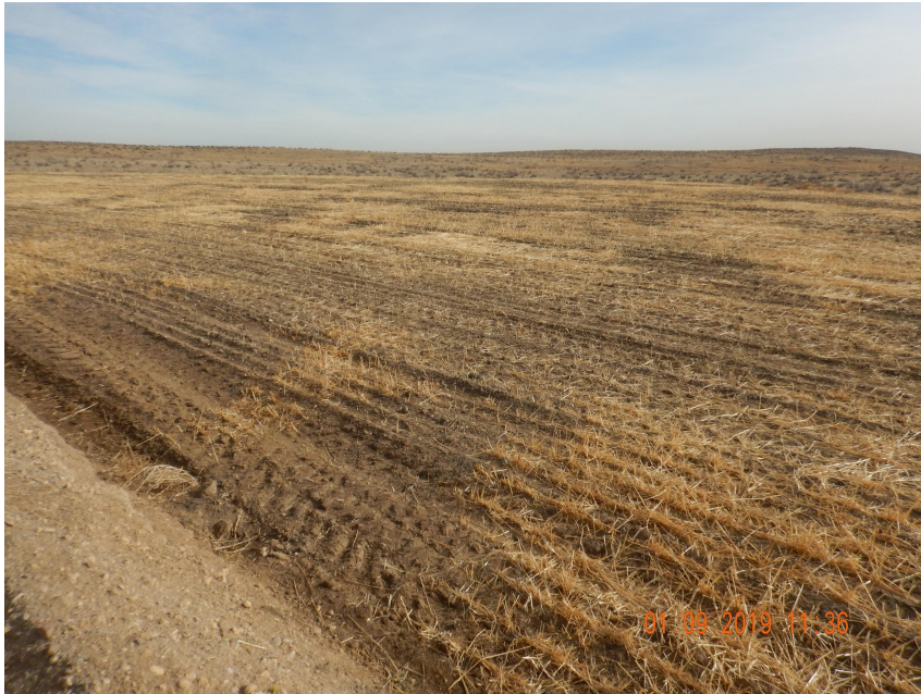
Photo 3. Photo taken from the eastern location, facing Northeast. Operator has performed interim reclamation activities with the evidence of drilling rows and straw crimped mulch. However, interim areas do not appear to be properly contoured to the surrounding landscape- see Photos 5 & 6.
