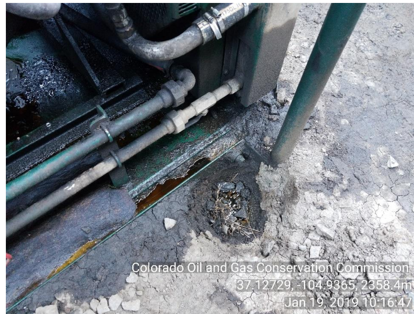
Photo 4 fluid and stained soil under drain plug of liquid ring skid
