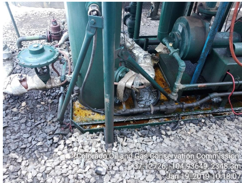
Photo 10 stained soil around liquid ring moto skid and trash in skid
