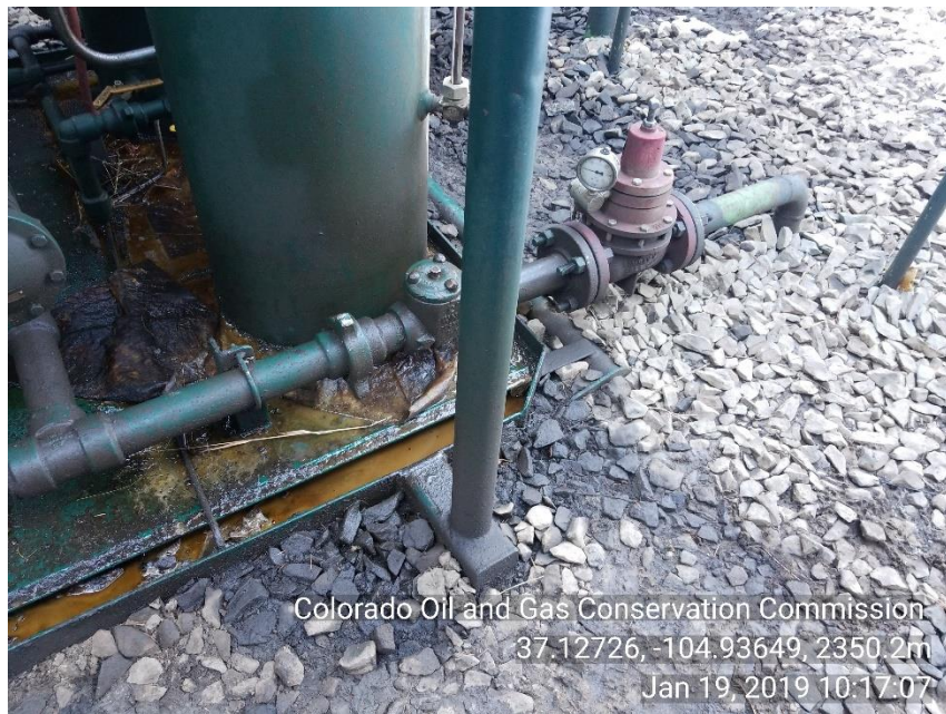
Photo 5 stained soil around liquid ring moto skid
