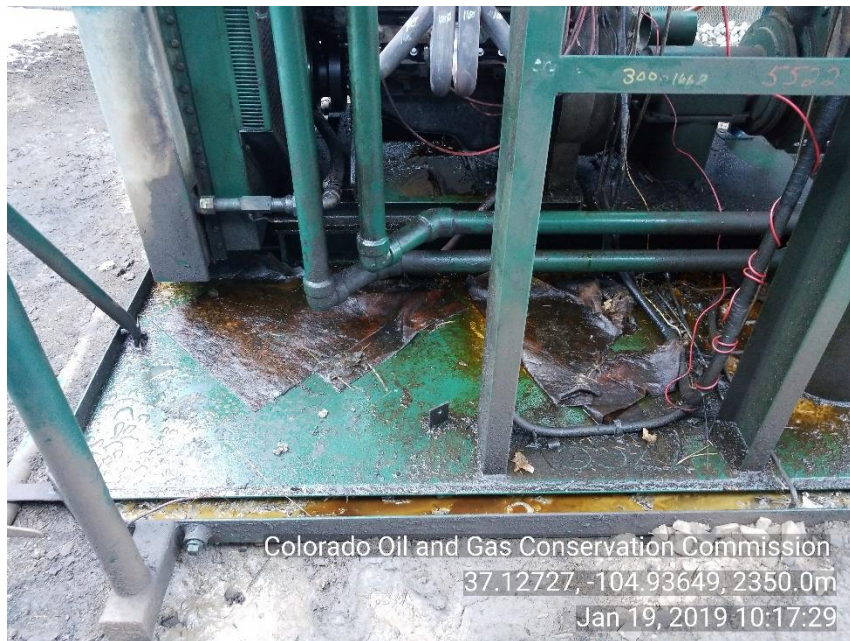
Photo 7 stained soil around liquid ring moto skid and trash in skid
