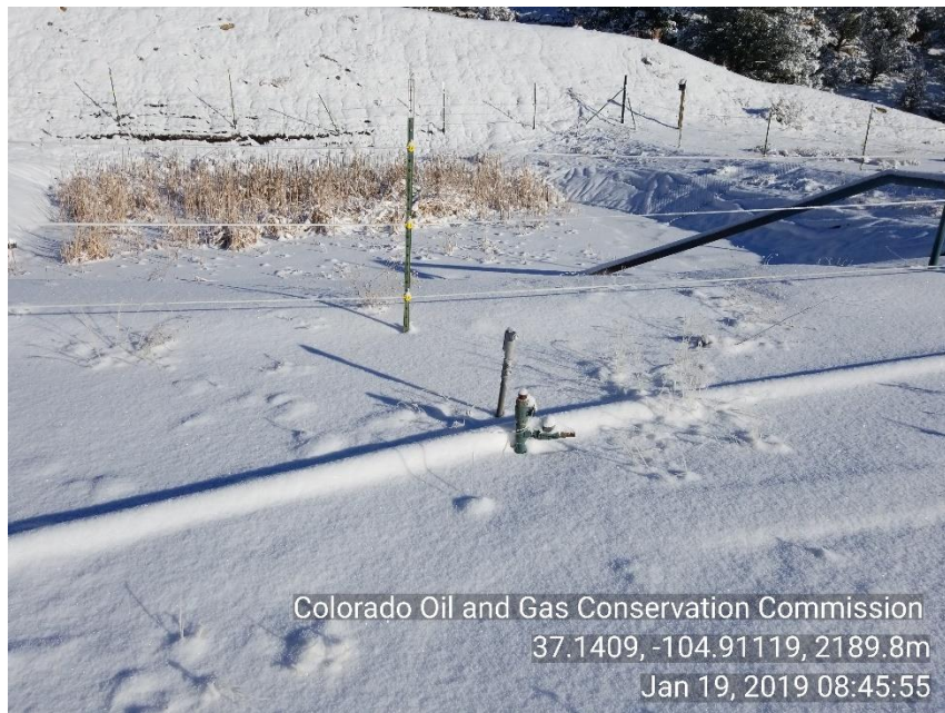
Photo 5 unused, unmarked and not LOTO riser
