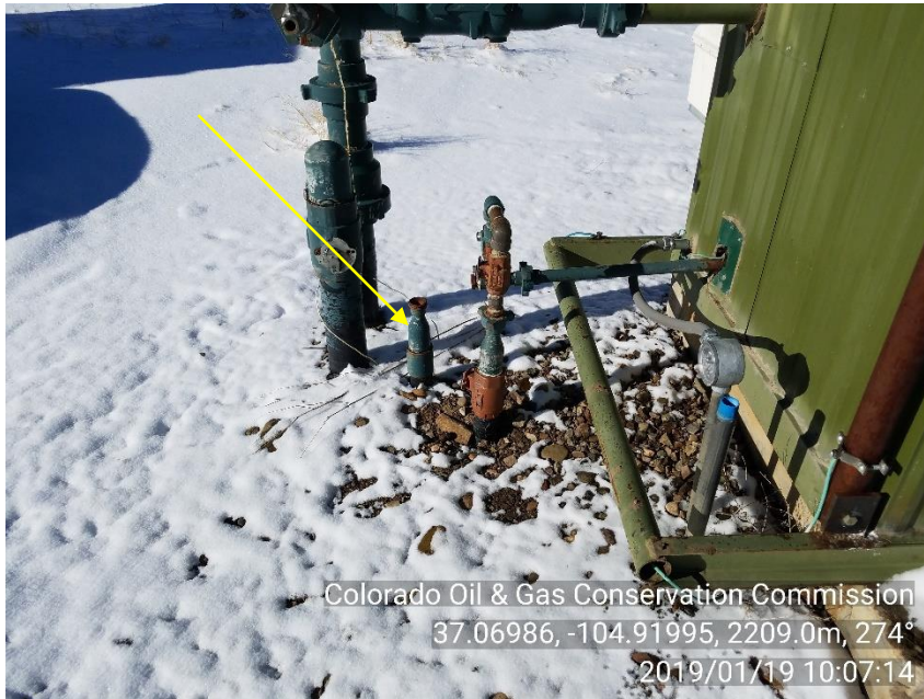
PHOTO 5: UNMARKED RISER WITH NO LO/TO
