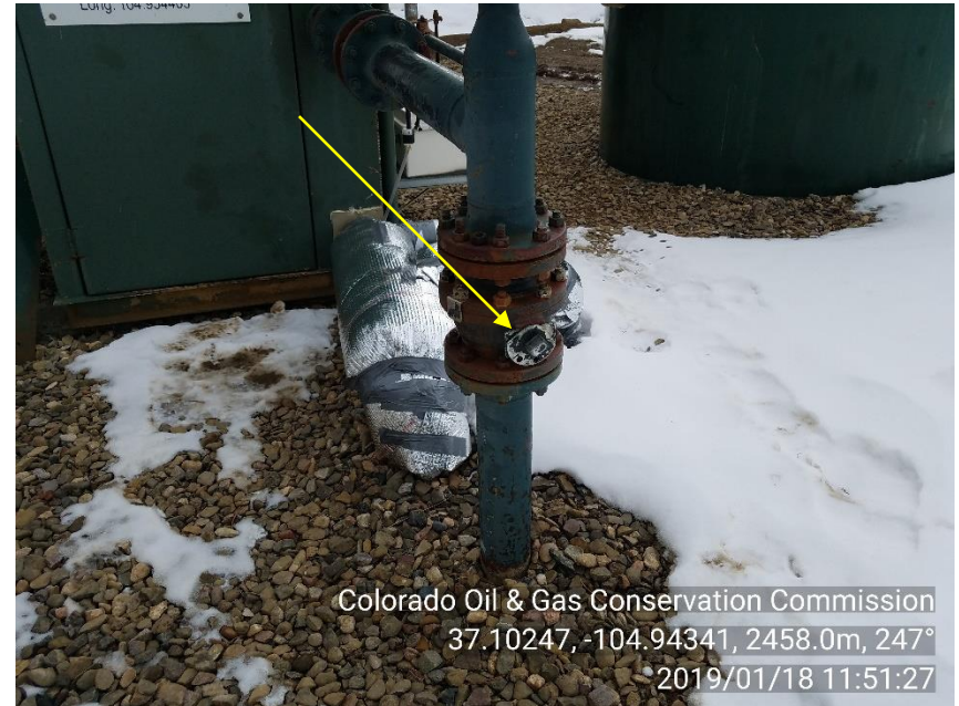
PHOTO 6: 3" VALVE ON SALES SIDE OF METER IS PINCHED BACK HALF WAY
