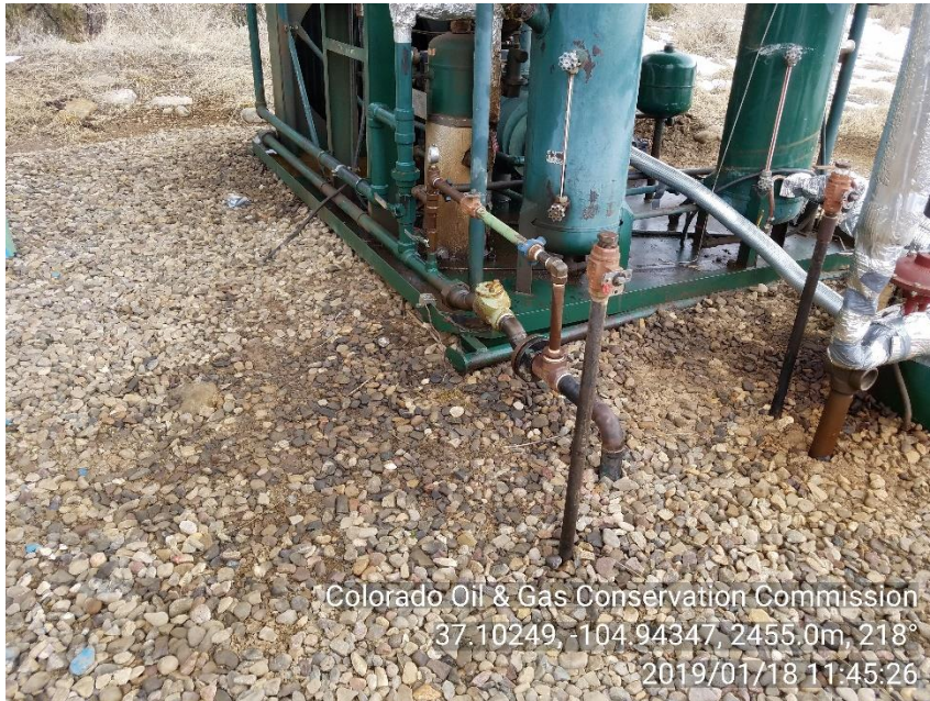
PHOTO 5: STAINED SOIL NEAR SCRUBBER DRAIN PLUG ON COMPRESSOR SKID
