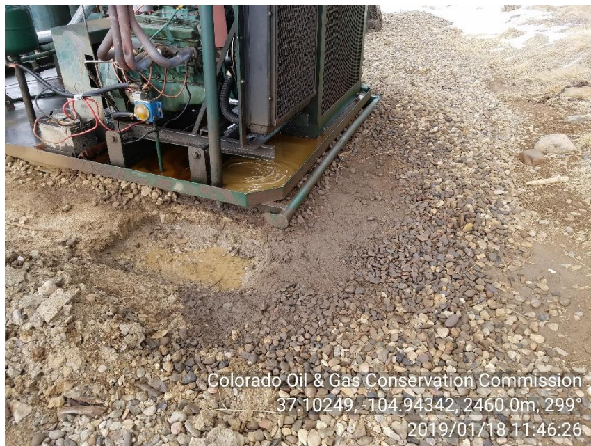
PHOTO 3: STAINED SOIL NEAR DRAIN PLUG ON COMPRESSOR SKID
