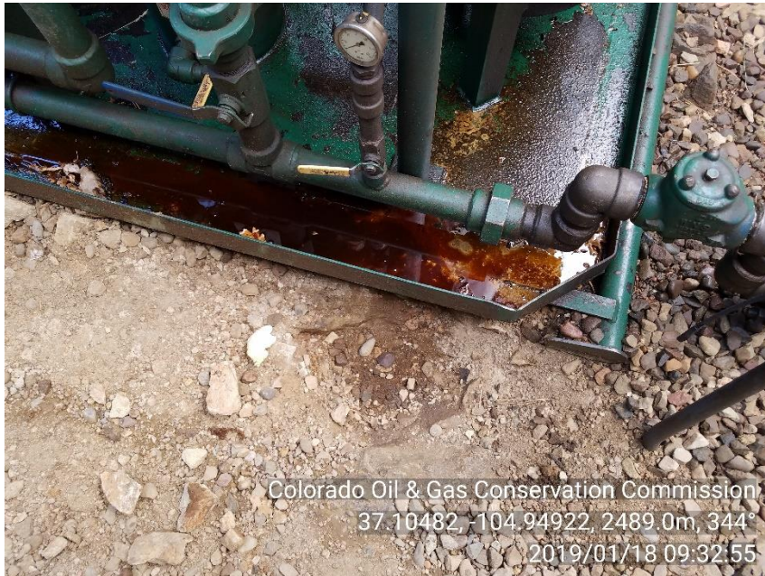
PHOTO 7: EXISTING HOLE NEAR COMPRESSOR SKID DRAIN PLUG APPEARS TO HAVE STAINED SOIL IN HOLE
