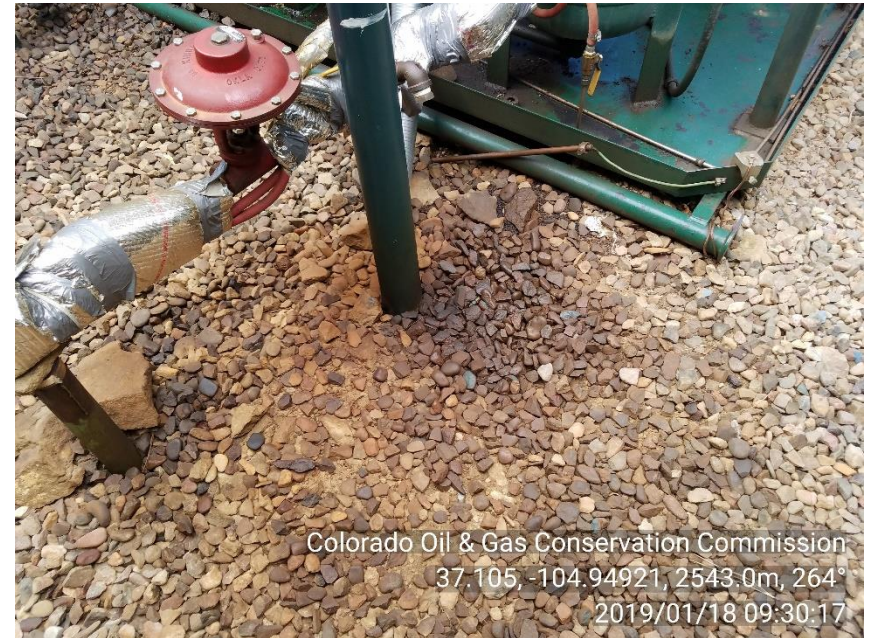
PHOTO 6: STAINED SOIL NEAR EXHAUST PIPE OF COMPRESSOR SKID
