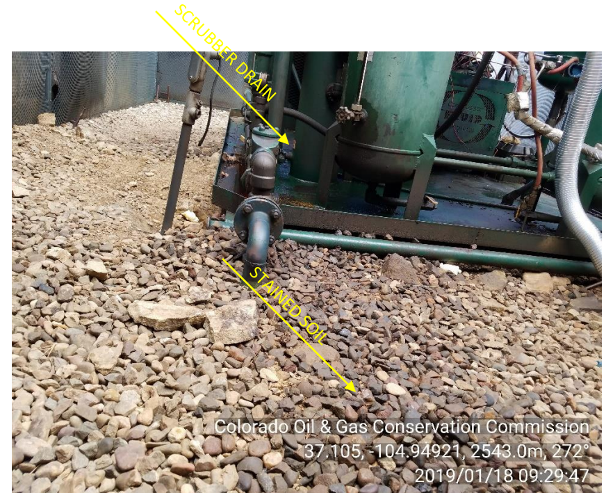
PHOTO 4: STAINED SOIL OUTSIDE OF COMPRESSOR SKID THAT APPEARS TO BE COMING FROM SCRUBBER DRAIN
