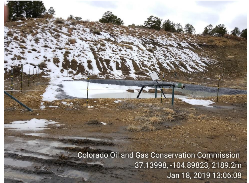
Photo 4 Electric fence around lined pit is in disrepair
