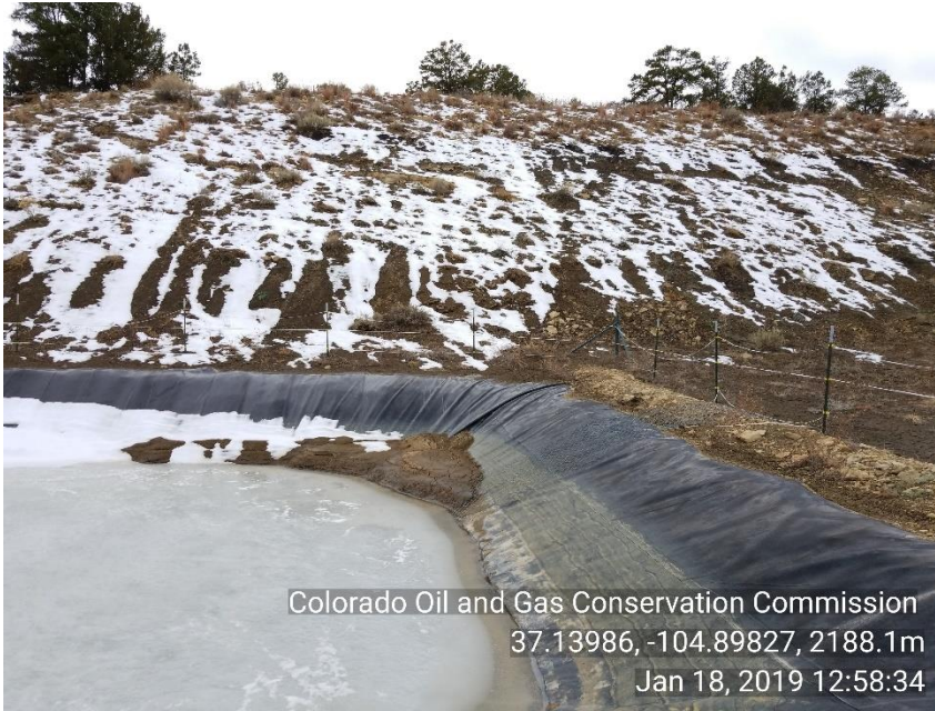
Photo 3 not proper BMP's Sediment is going in lined pit
