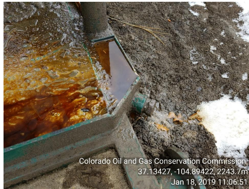
Photo 4 stained soil and fluid dripping out of liquid ring skid
