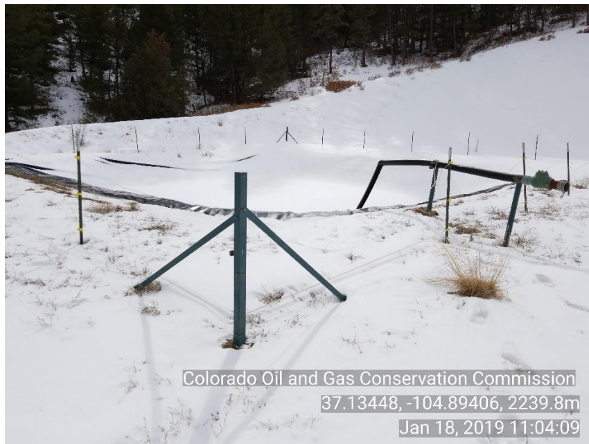
Photo 9 electric fence around lined pit in disrepair
