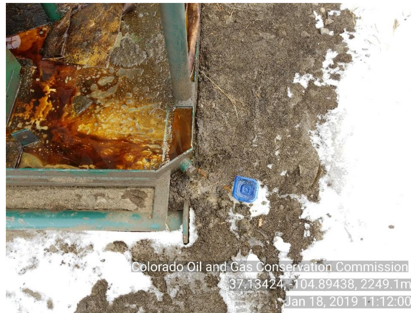
Photo 8 soil sample taken where fluid is dripping out of skid
