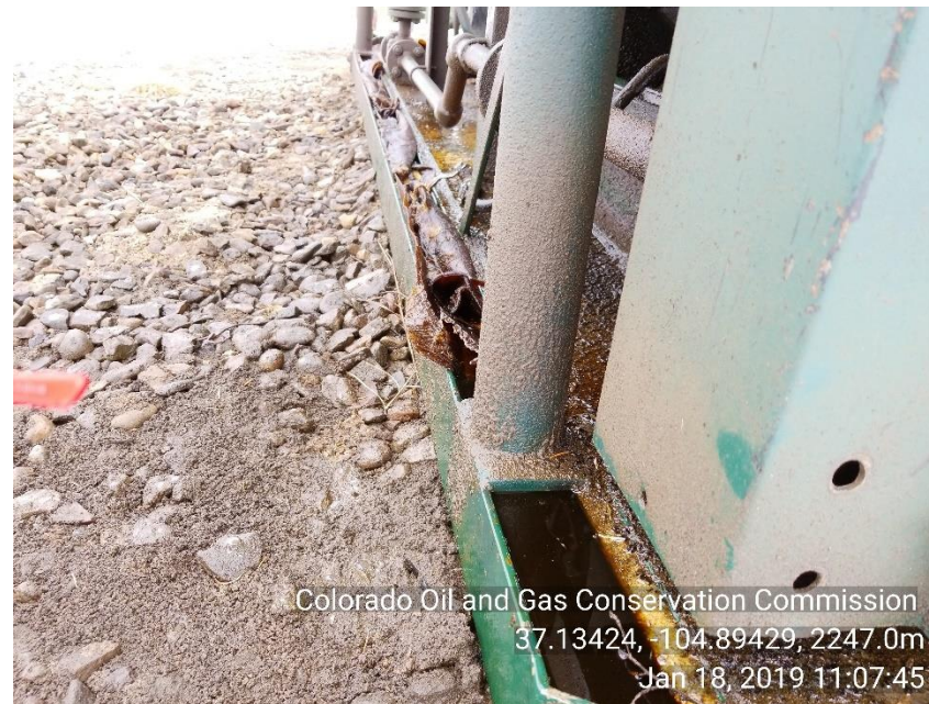
Photo 6 stained soil and fluid dripping out of liquid ring skid
