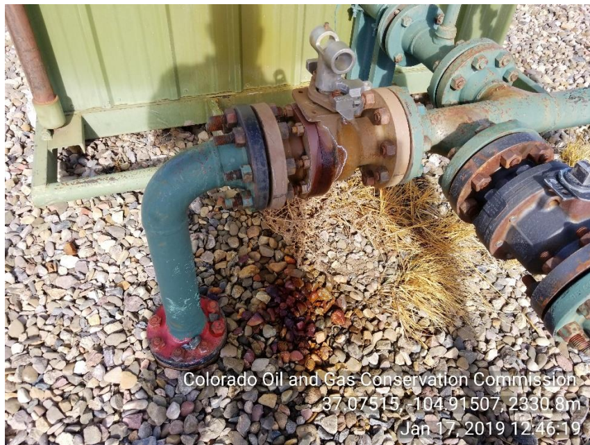
Photo 3 VLV leaking at time of inspection
