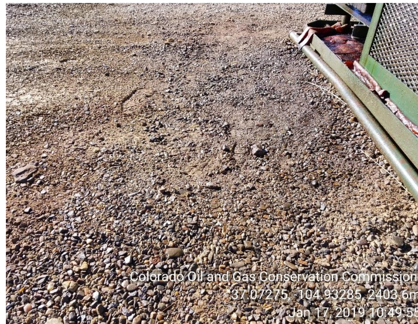
Photo 2 stained soil around liquid ring compressor
