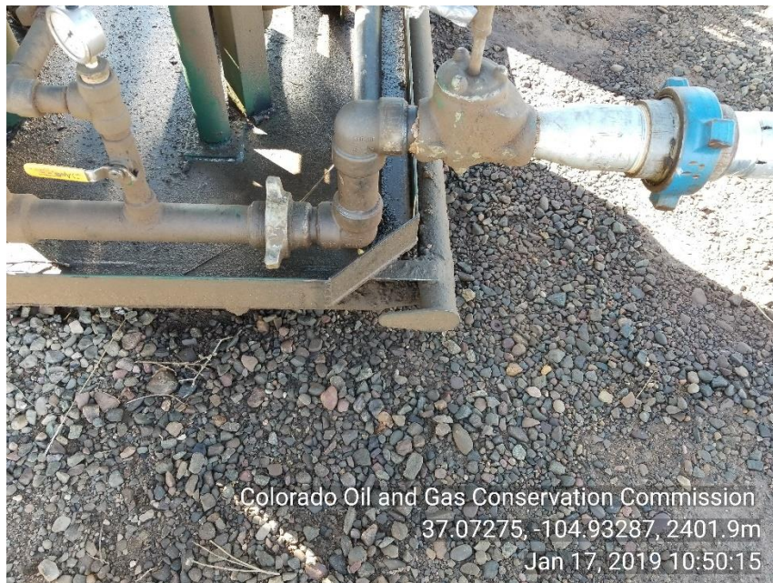
Photo 3 Stained soil around liquid ring compressor
