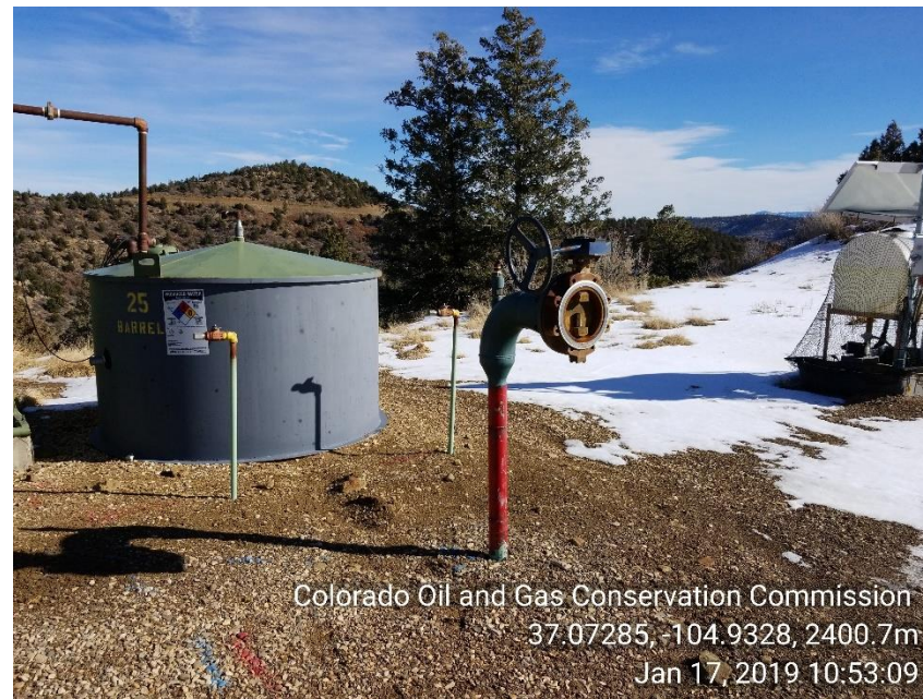
Photo 8 Unused, unmarked and not LOTO risers
