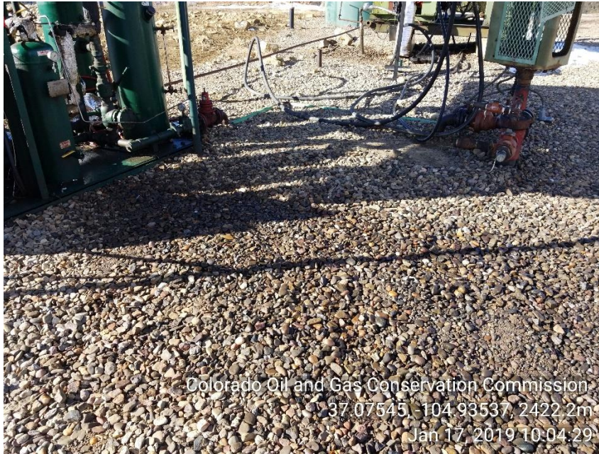
Photo 3 Stained soil around liquid ring and WH
