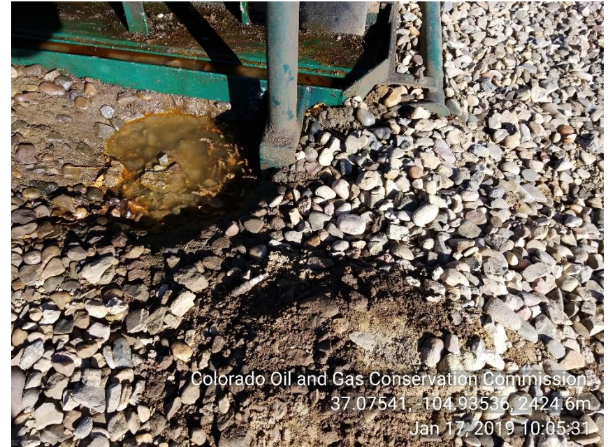
Photo 6 Stained soil around drain plug of liquid ring
