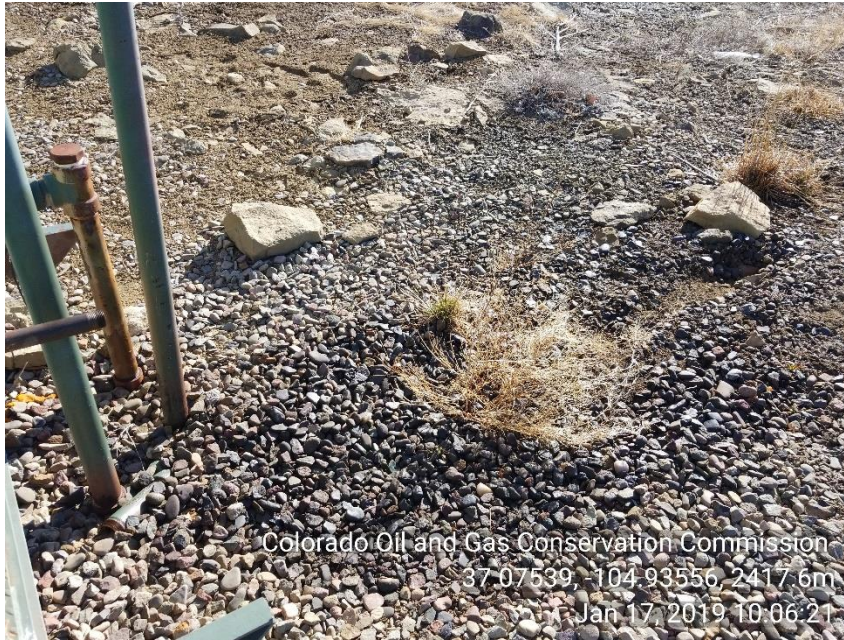
Photo 7 stained soil under 1" drain line from separator
