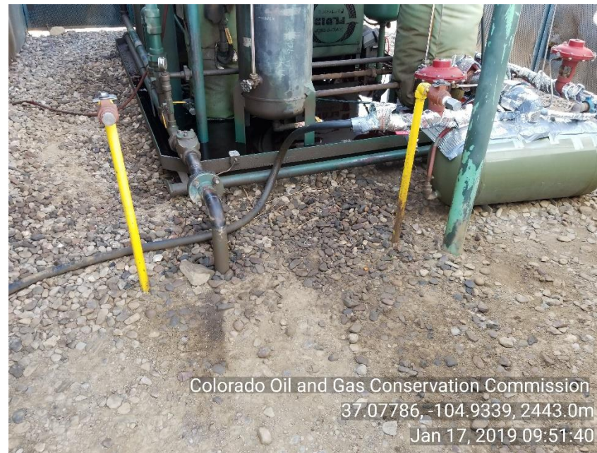
Photo 4 Stained soil around liquid ring compressor
