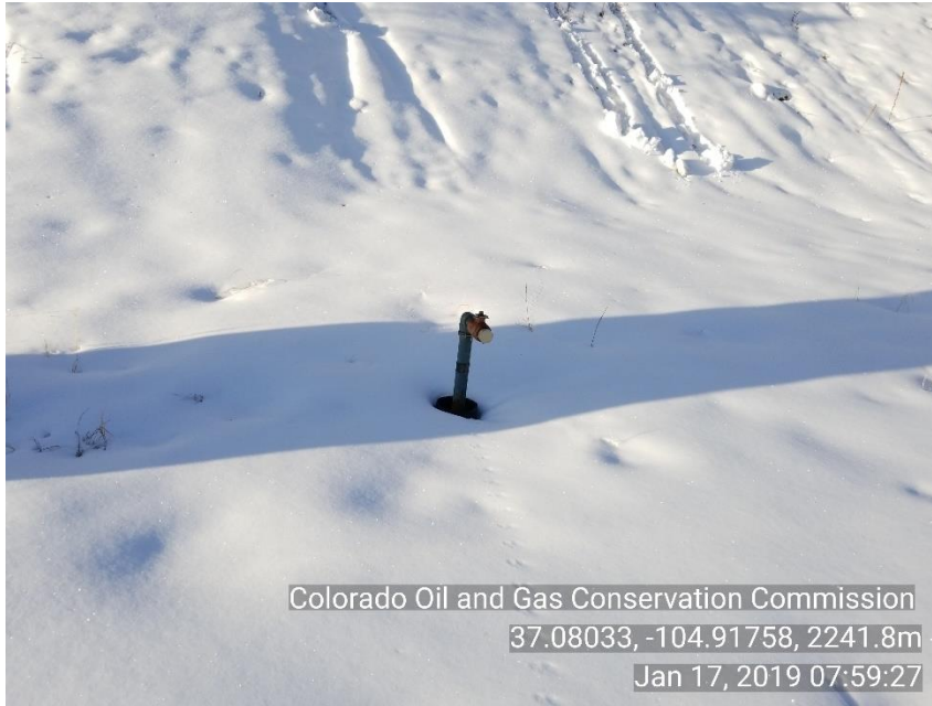
Photo 3 Unused, unmarked riser not LOTO
