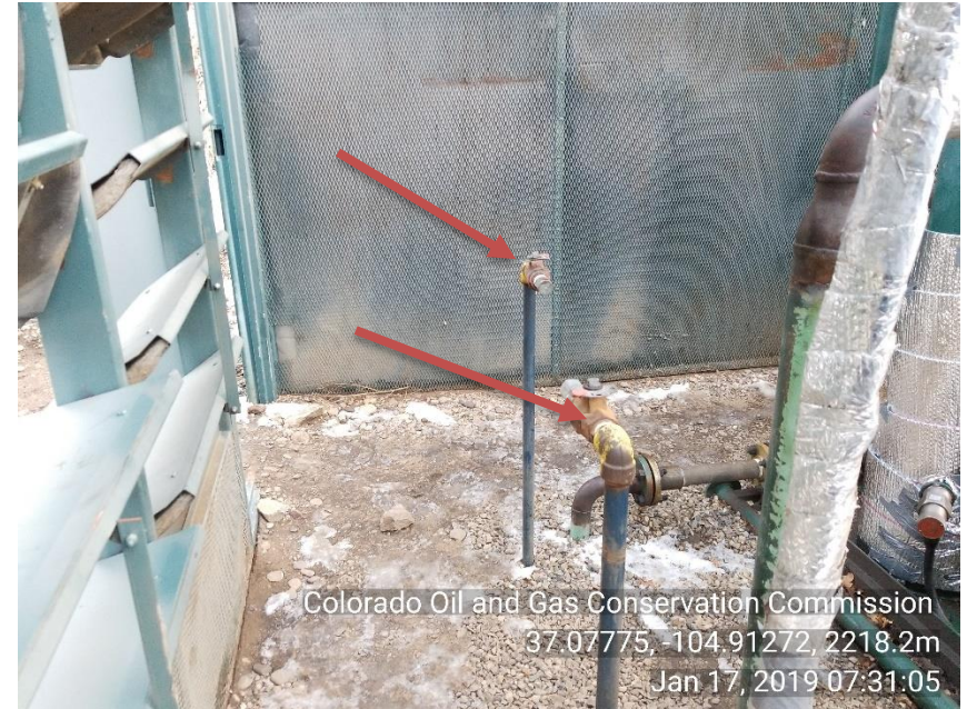
Photo 4 Unmark and unused risers not LOTO
