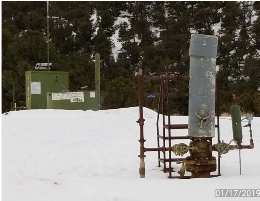
Photo 1. Location looking southwest.
