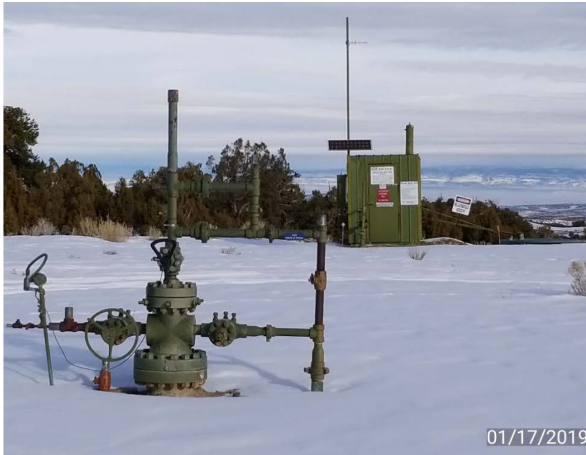
Photo 1. Location looking north.
