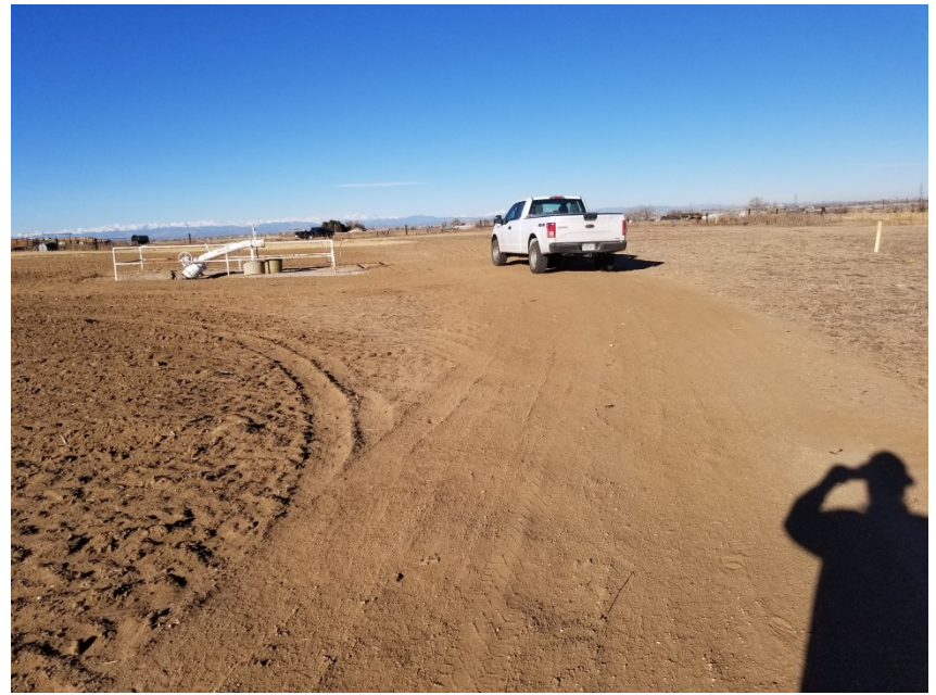
Photo 4. Photo taken from the access road looking into the location, facing West. See comments from Photo 1.
