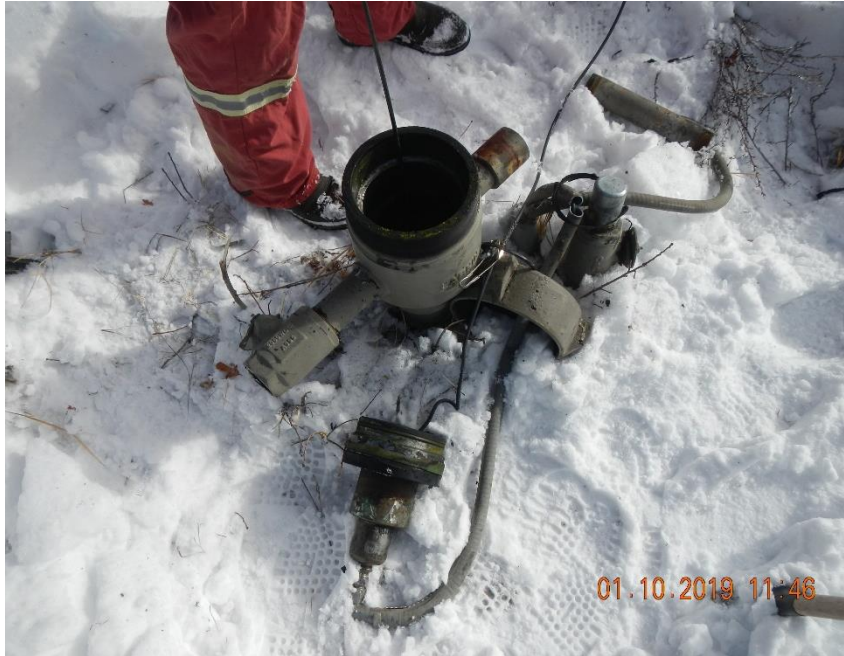
Removing rugged cable from well bore.
