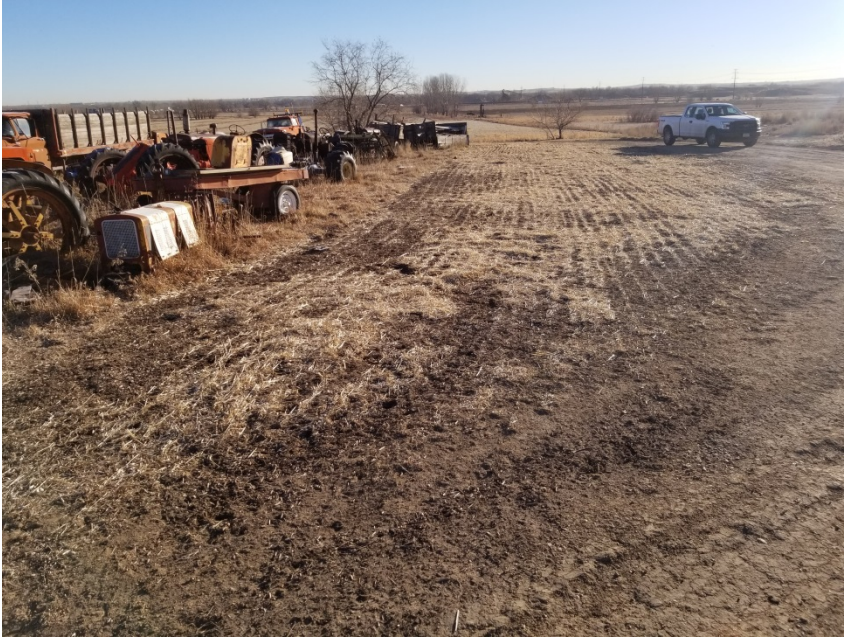
Photo 1. Photo taken from the well location looking towards the facility, facing East. Appears the Operator has performed final reclamation activities on the well location and the facility, with the evidence of drilling rows and straw crimped mulch.
