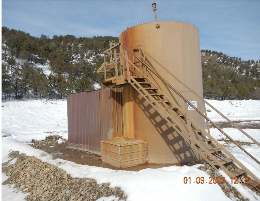
Rust colored staining on AST and adjacent equipment.
