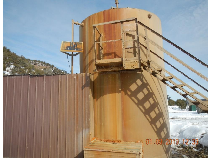
210 bbl. AST and associated equipment are stained with rust colored residue.
