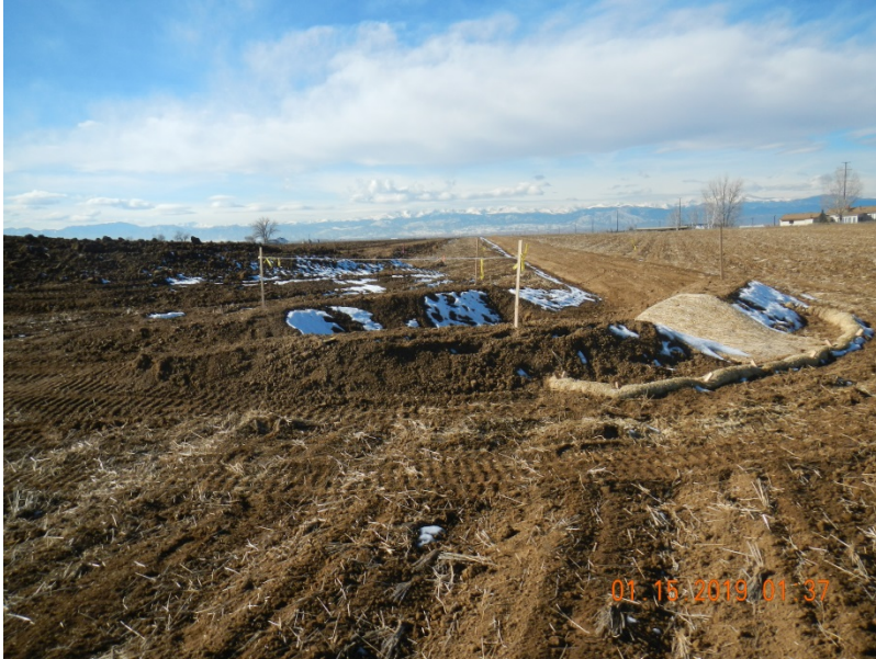
Photo 3. Photo taken from the northeastern perimeter of the location, facing West. Operator has installed a sediment trap with a temporarily stabilized outlet. See comments from Photo 1.
