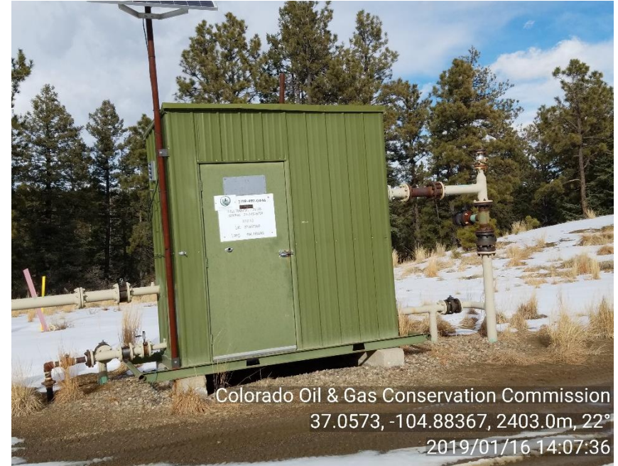
PHOTO 2: WELL SIGN/METER HOUSE
