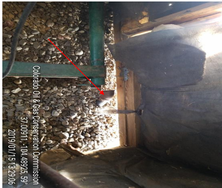
PHOTO 5: UNMARKED UNUSED RISER/ NO PLUG
