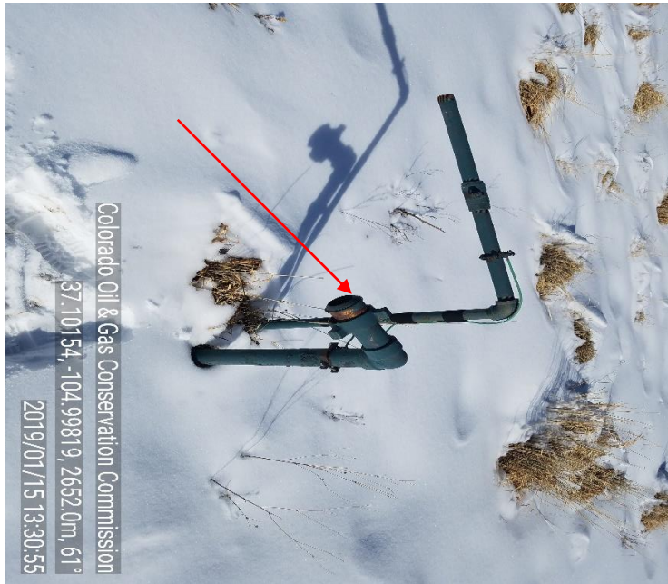
PHOTO 7: UNMARKED UNUSED RISER/ NO PLUG
