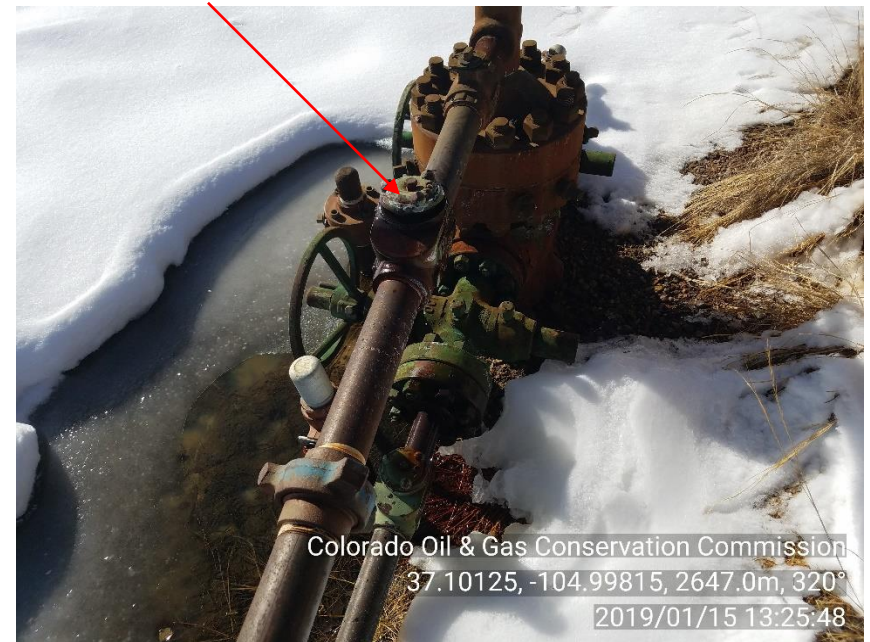
PHOTO 4: CHECK VALVE BROKE LEAKING CLEAR FLUID
