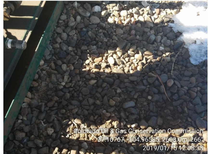
PHOTO 4: STAINED SOIL NORTH SIDE OF COMPRESSOR SKID UNDER DRAIN PLUG
