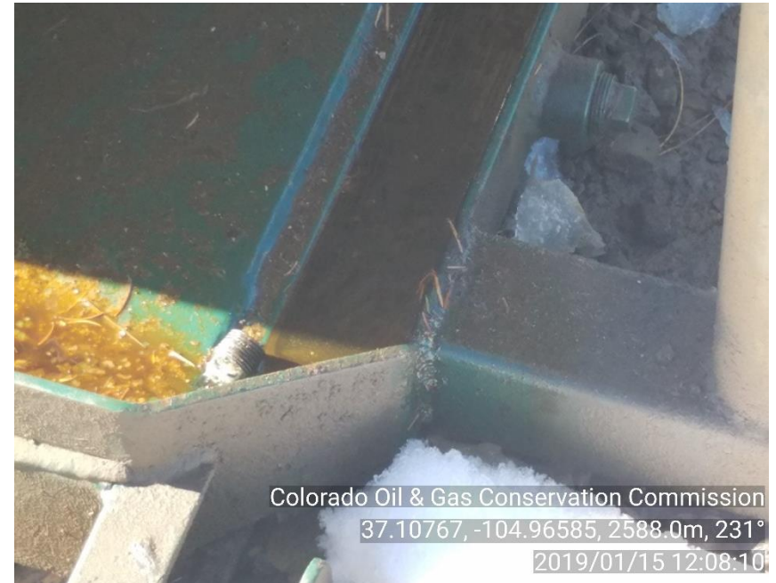
PHOTO 2: SKID CONTAINMENT IS FULL OF FLUID AND RUNNING OVER
