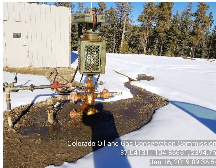
Photo 2 WH packing leaking
