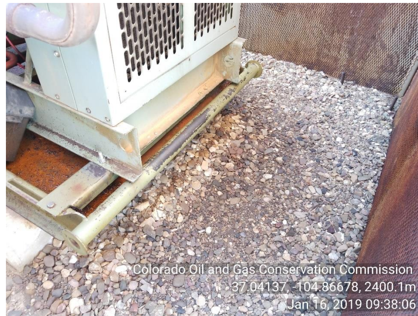
Photo 6 Stained soil around motor skid
