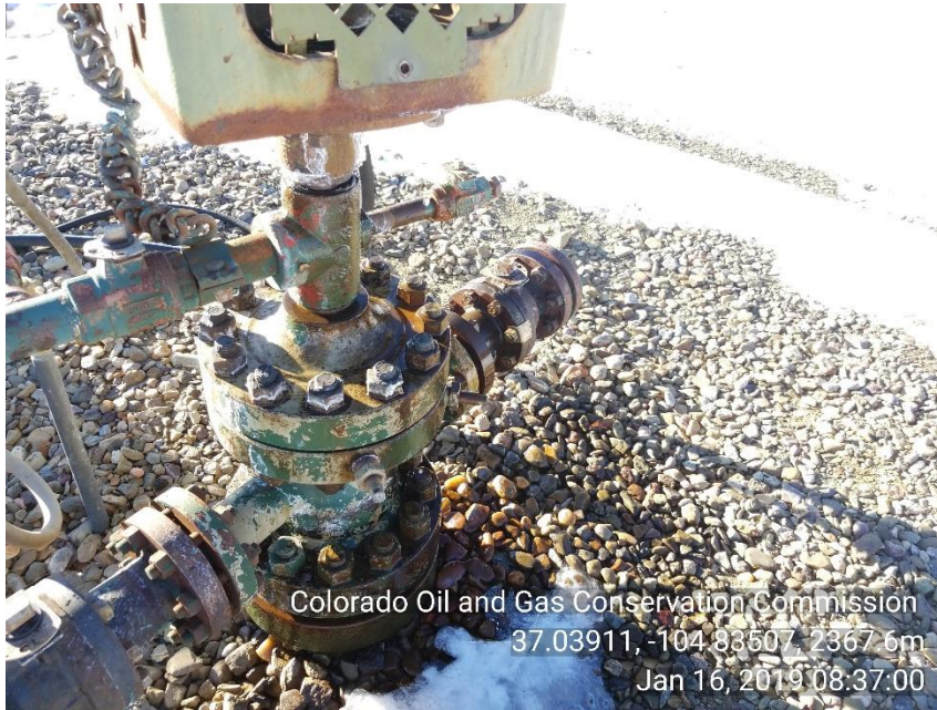
Photo 3 Packing on well head leaking
