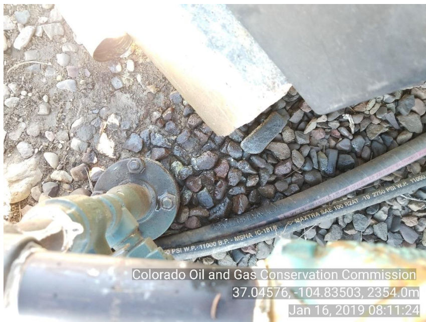
Photo 3 Stained soil around 1" fuel gas line
