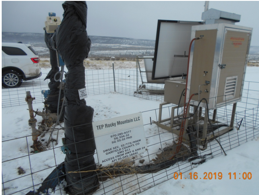
Wellhead with line heater.
