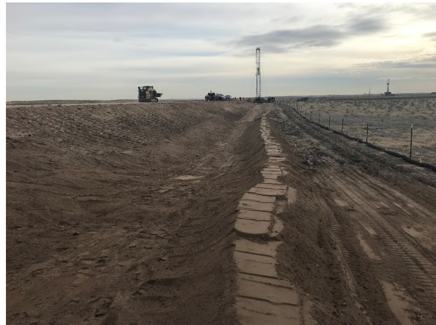
Photo NBL10. Ripping and Filtrexx installed along eastern perimeter. Note: photo includes a sediment trap that is under construction.
