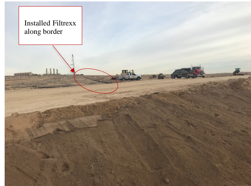
Photo NBL9. Filtrexx installed to enclose northern perimeter. A sediment trap is under construction in the foreground.
