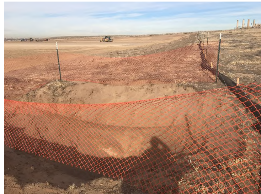
Photo NBL5. Photo displays restoration of gap in Filtrexx perimeter.
