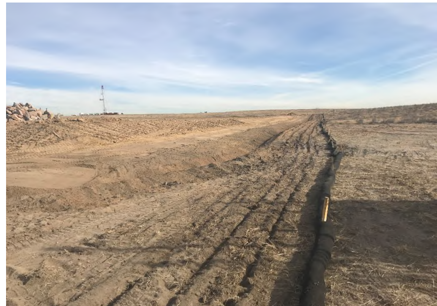
Photo NBL1. Perimeter ripping has been implemented and Filtrexx properly reinstalled.
