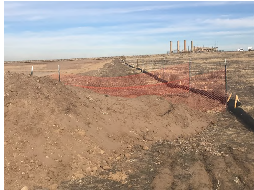
Photo NBL4. Photo displays restoration of gap in Filtrexx perimeter.
