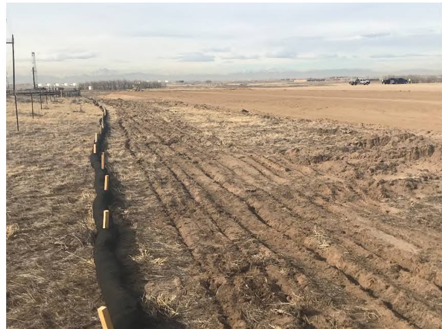
Photo NBL2. South perimeter ripping has been implemented and Filtrexx properly reinstalled.
