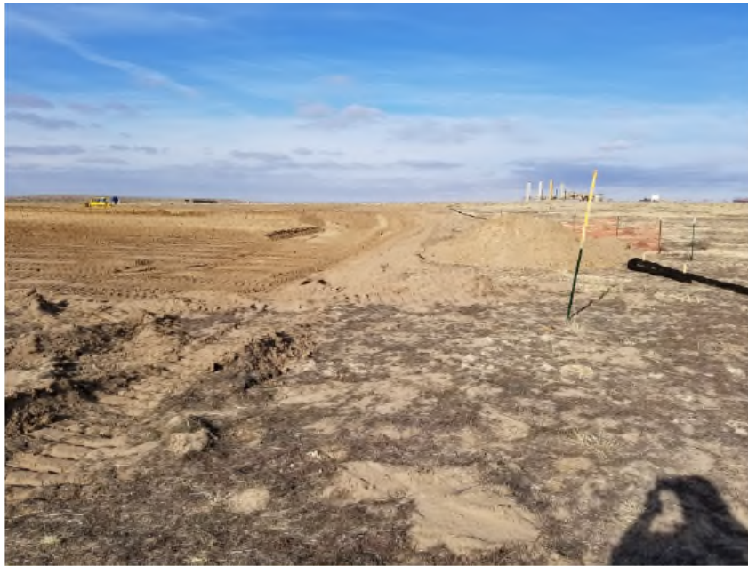
Photo 3. Photo taken from the southeastern perimeter of the location, facing North. Photo depicts breaks in the perimeter of the filtrex BMP.
