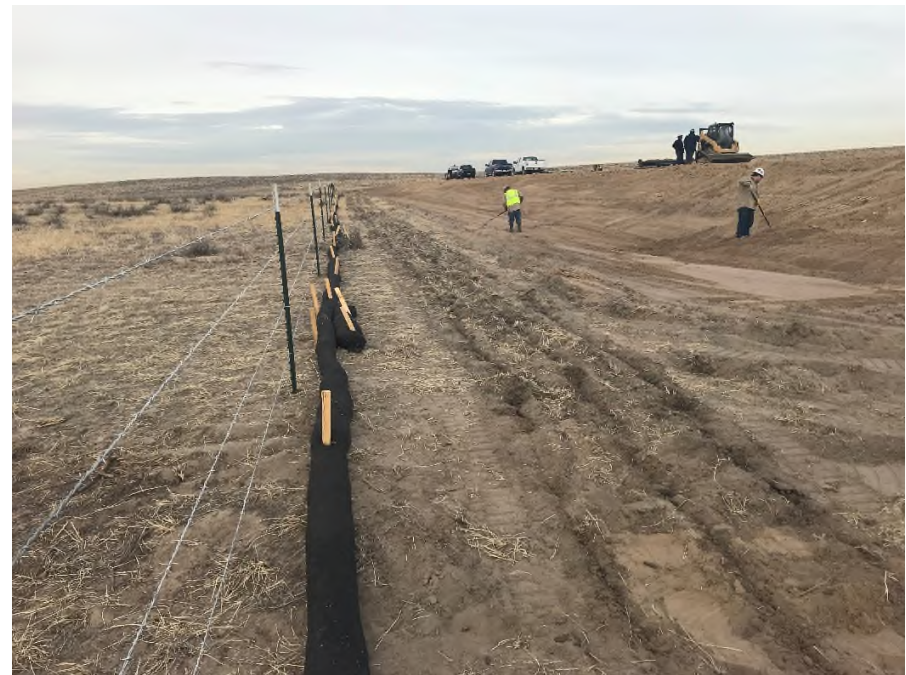
Photo NBL14. Ripping was added to the southwestern perimeter. Filtrexx remains and is properly maintained.
