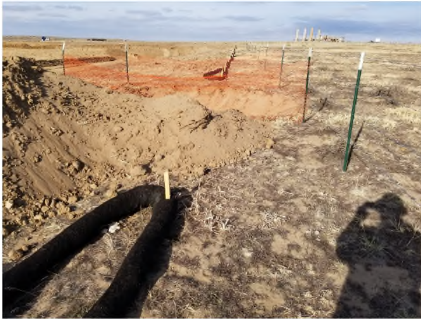
Photo 4. Photo taken from the Eastern perimeter of the location, facing North. Photo depicts breaks in the perimeter of the filtrex BMP adjacent to open fenced pothole.
