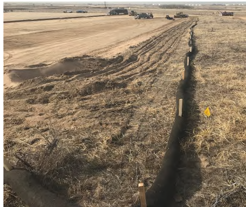
Photo NBL7. Filtrexx installed to close north perimeter break.
