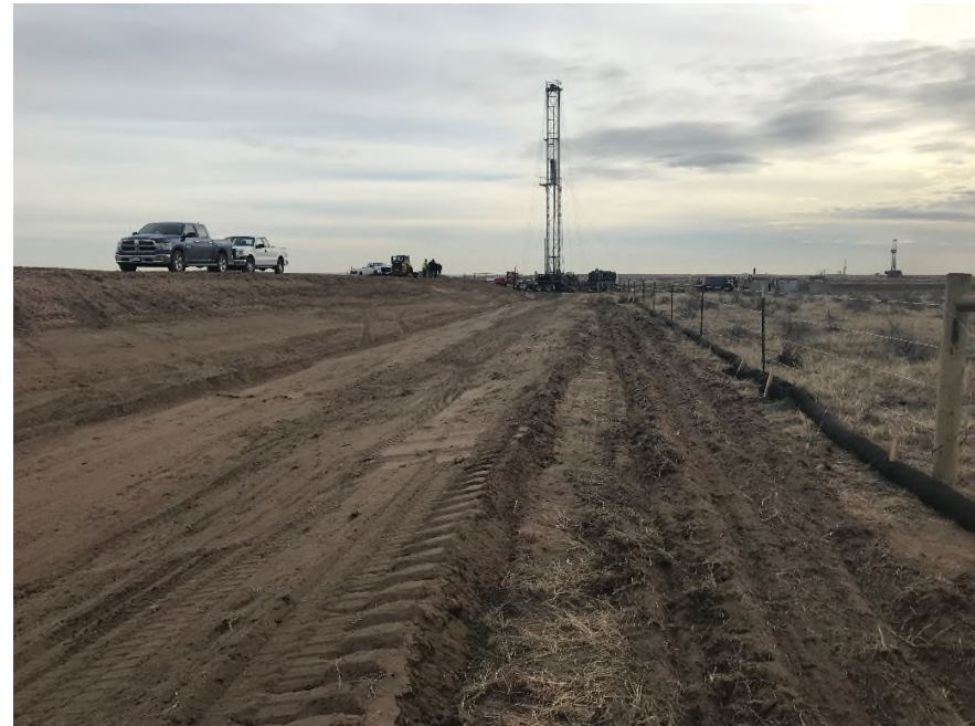
Photo NBL11. Ripping and Filtrexx BMPs installed along western perimeter.
