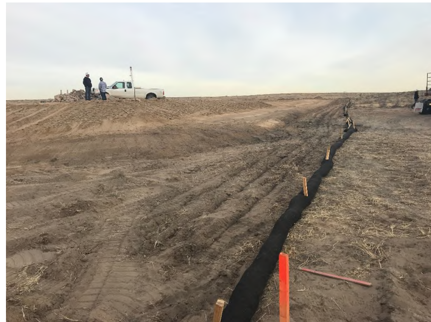
Photo NBL13. Perimeter ripping and Filtrex installed along southern perimeter.
