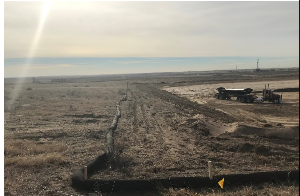
Photo NBL8. Filtrexx installed to close east perimeter break.
