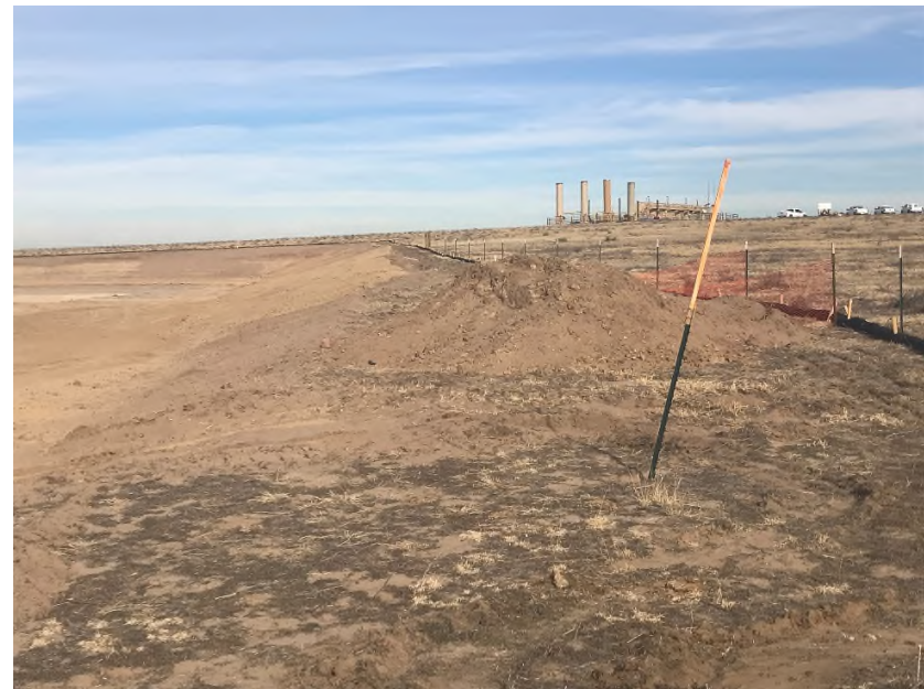
Photo NBL3. Additional Filtrex has been installed to the east perimeter to fill breaks.
