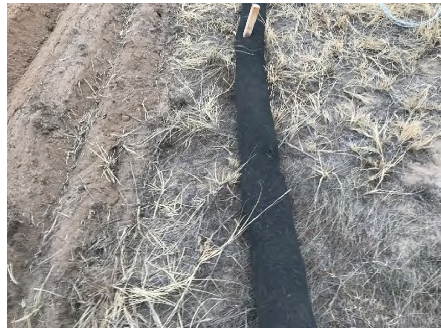
Photo NBL12. Damaged Filtrexx along western perimeter replaced.
