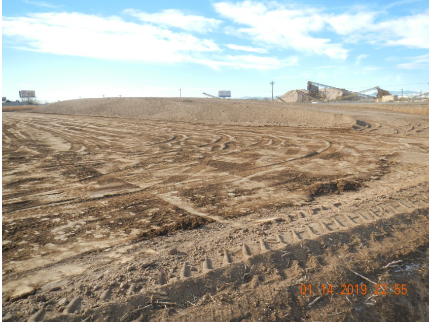
Photo 9. Photo taken from the northern perimeter of the location. The topsoil stockpile being stored along the western area has been temporarily stabilized with equipment tracking.
