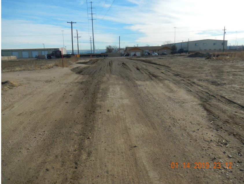
Photo 11. Photo taken from the entrance of the location off CR 27, facing North. Appears Operator has not installed any tracking device or gravel to potentially limit tracking onto the county road.
