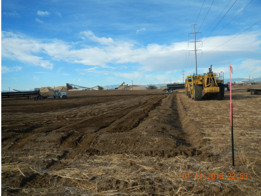
Photo 1. Photo taken from the northeastern perimeter of the location, facing West. Photo illustrates a ditch and berm BMP that has been installed around the perimeter of the location.
