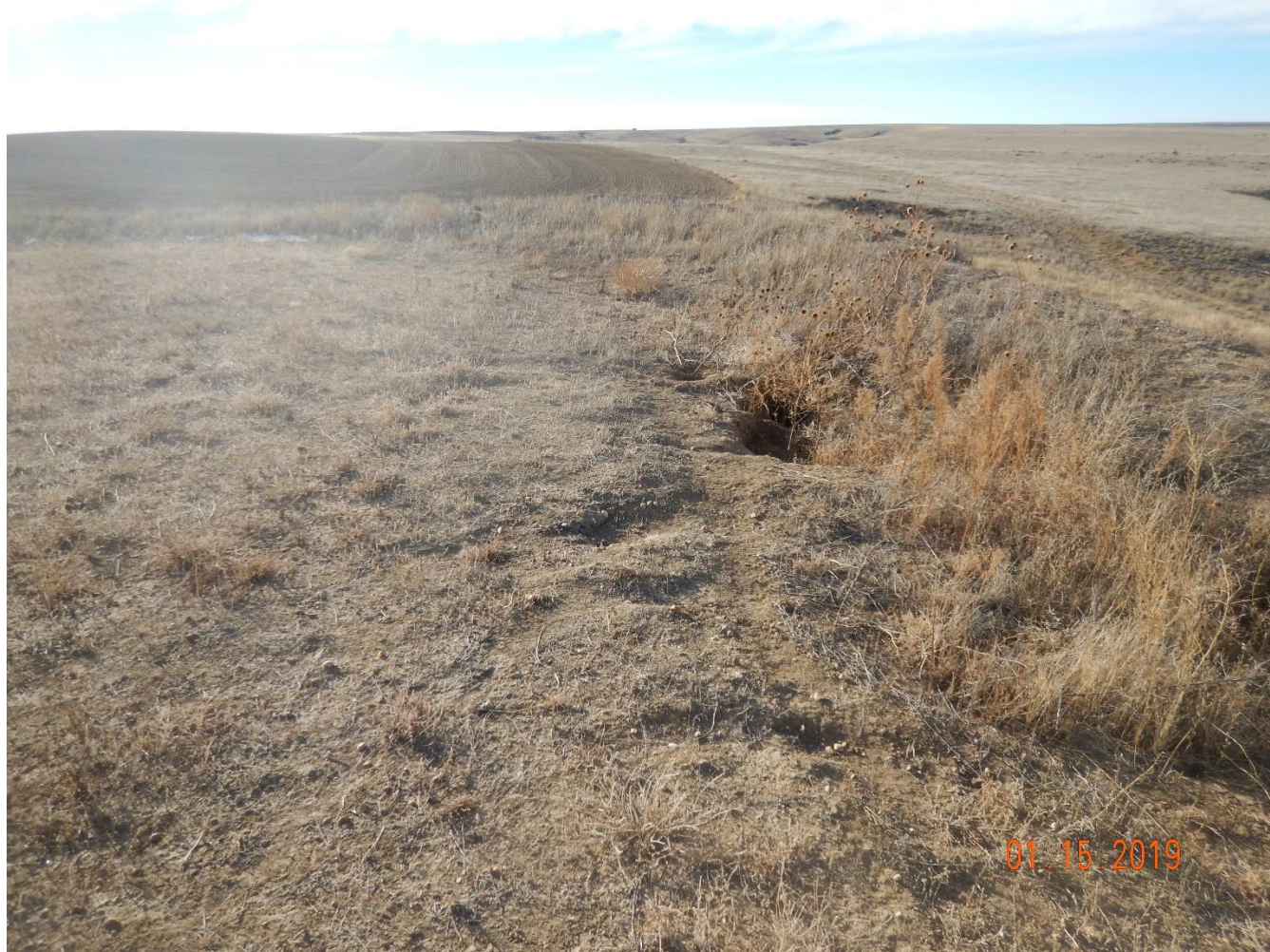
Photo 8: Photo taken from the ditch on the southwest corner of the location, facing south. Previous inspections documented that stormwater runoff has incised the ditch along the west end of the pad and created sinkholes within the ditch. Photo shows a new sinkhole has developed within the ditch.
