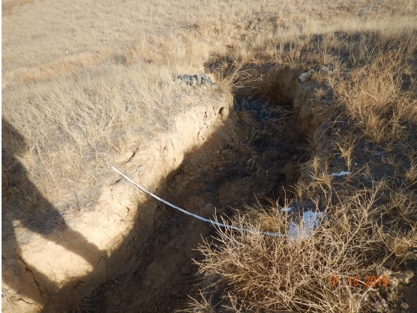
Photo 20: Photo taken from the gully on the northwest end of the pad, facing north. Photo shows gully erosion has not been repaired/stabilized. 6 foot measuring stick for reference.
