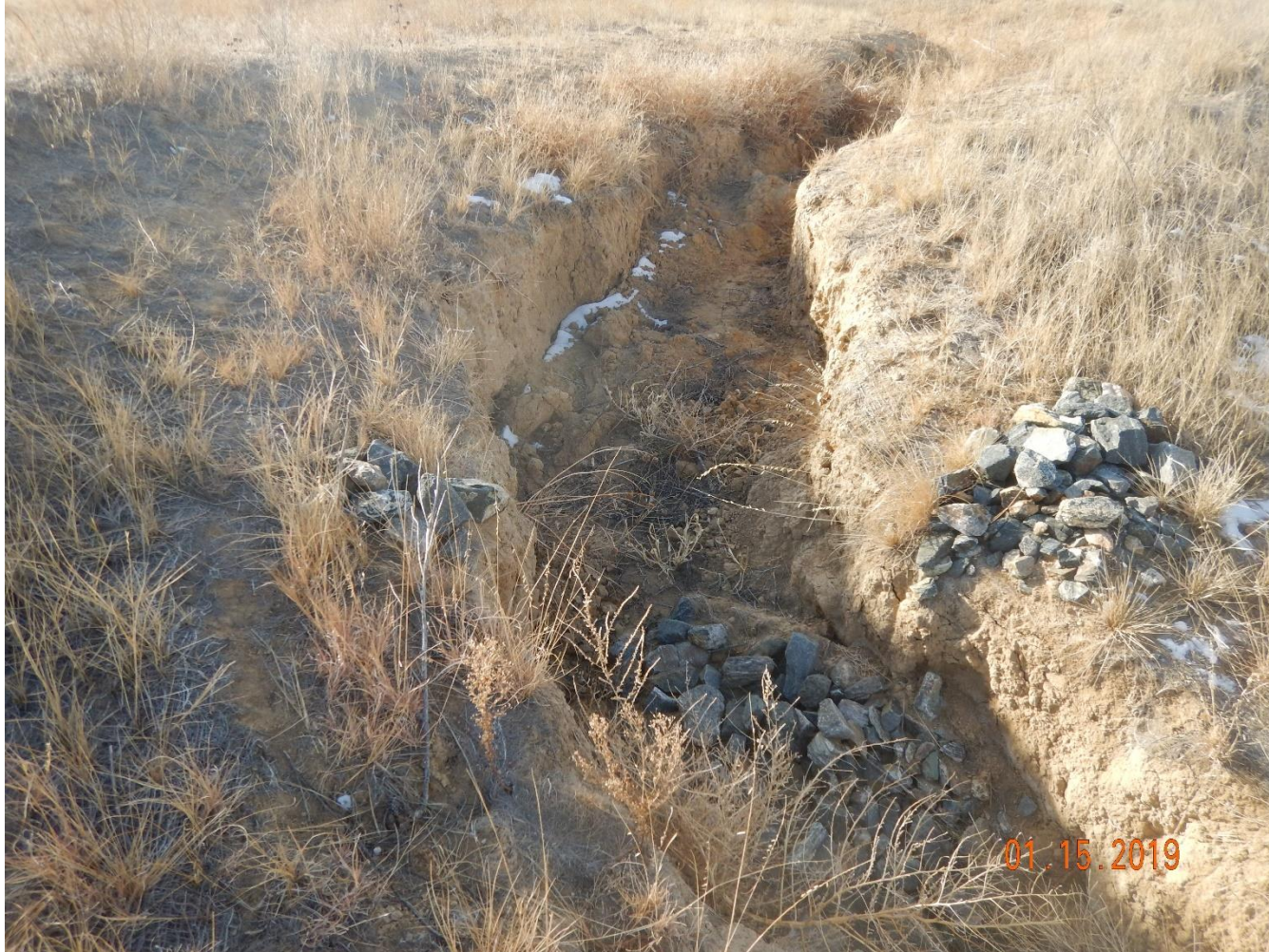
Photo 21: Photo taken from the gully on the northwest end of the pad, facing southwest. Photo shows gully erosion has not been repaired/stabilized.
