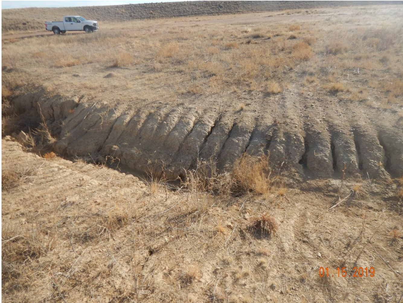
Photo 18: Photo taken from the ditch on the northwest end of the pad. Photos show stormwater runoff from the pad into the ditch has created rill erosion. Stormwater degradation has not been repaired or stabilized.
