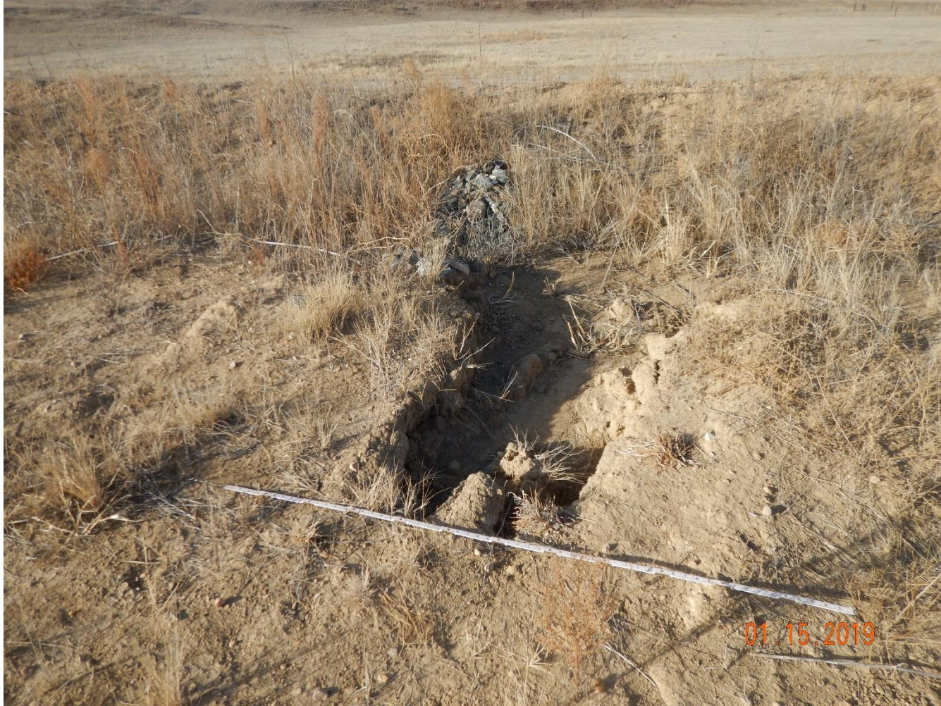
Photo 16: Photo taken from the ditch on the northwest end of the location, facing west. Photo shows erosion degradation cutting eastward into the pad has not been repaired or stabilized. 6 foot measuring stick for reference.
