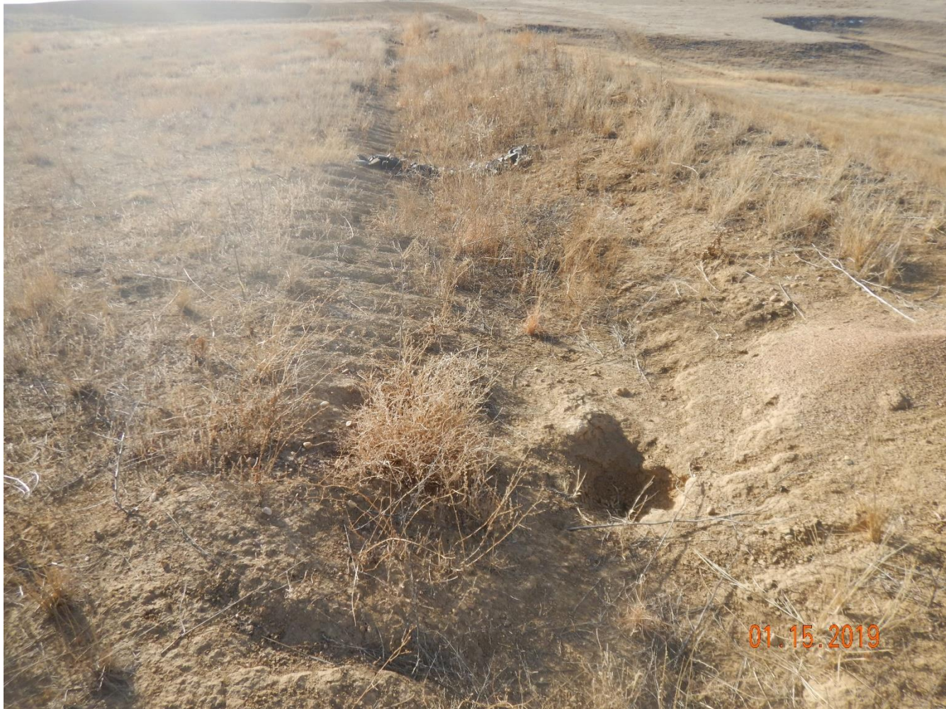
Photo 14: Photo taken ~100 feet north from photo 13. Photo shows a third sinkhole appears to be forming within the ditch along the west end of the location.
