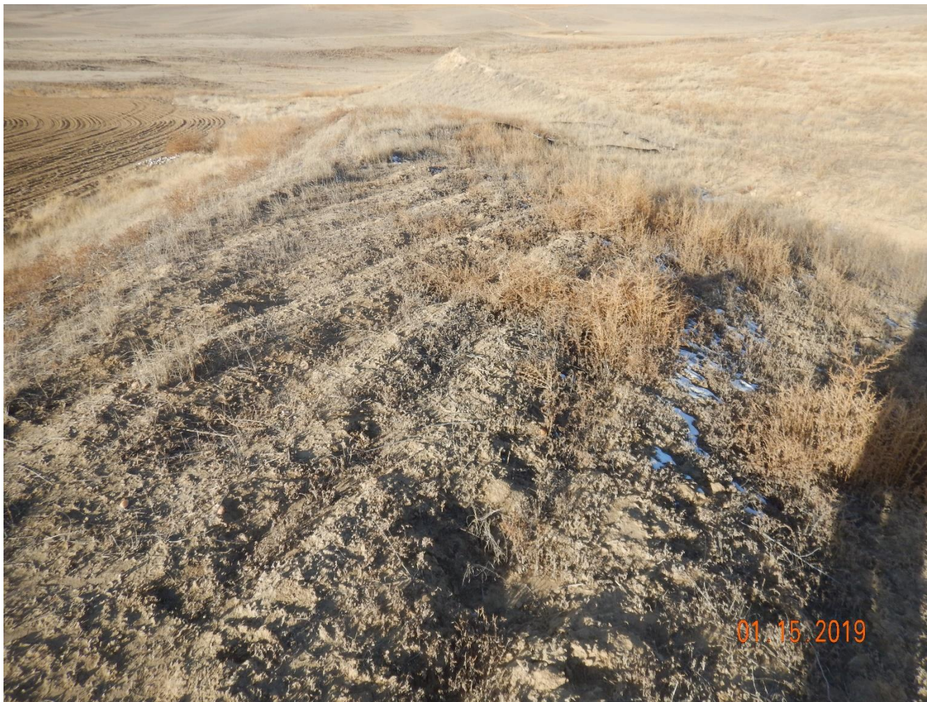
Photo 6: Photo taken from area of the “spoils” stockpile on the south end of the location, facing west. Photo shows areas of bare and exposed soil with large furrows. Previous inspections required operator to repair erosion and stabilize slopes. Photo shows erosion has not been repaired and BMPs have not been installed. Photo also show reclamation activities do not appear to have been conducted per CAs and COAs
