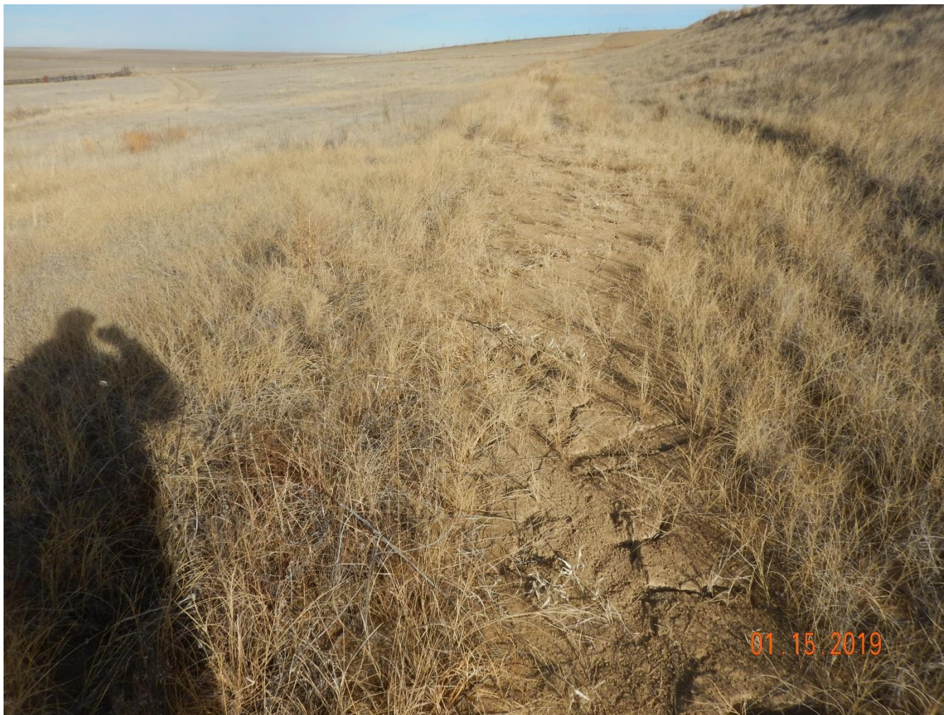
Photo 22: Photo taken from the stormwater ditch along the perimeter of the west end of the location. Previous inspection documented that ditch BMP has filled with sediment and is not longer in proper functioning condition. BMP should have been reclaimed during interim reclamation. Photo shows BMP remains filled with sediment. Photo also shows interim reclamation to reduce the area of disturbance has not been conducted.
