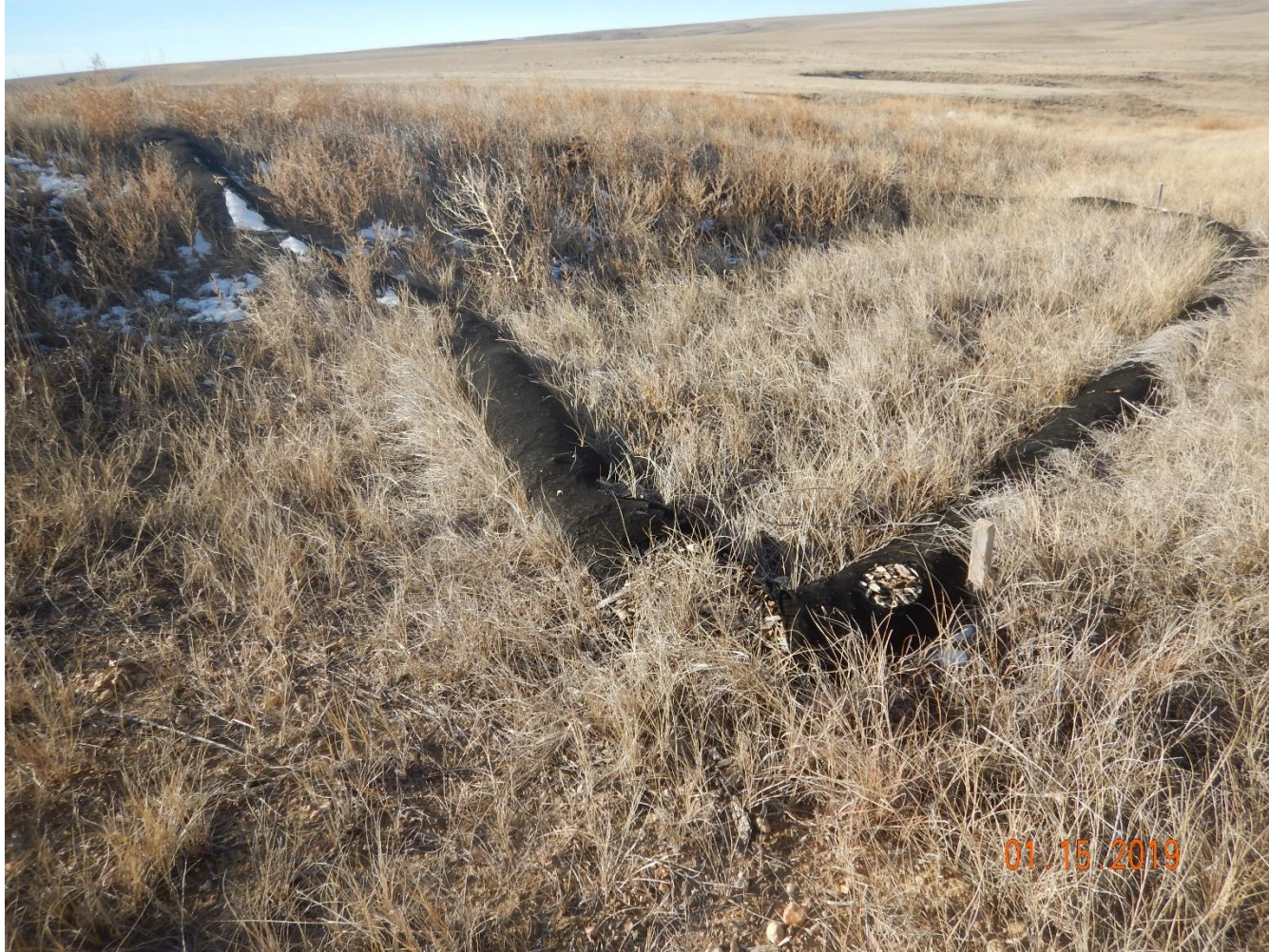
Photo 7: Photo taken from the south end of the location, facing southwest. Photo shows wood-mulch wattle stormwater ponding BMP. Previous inspection documented BMP was degrading. Photo shows BMP has not been maintained/repaired.
