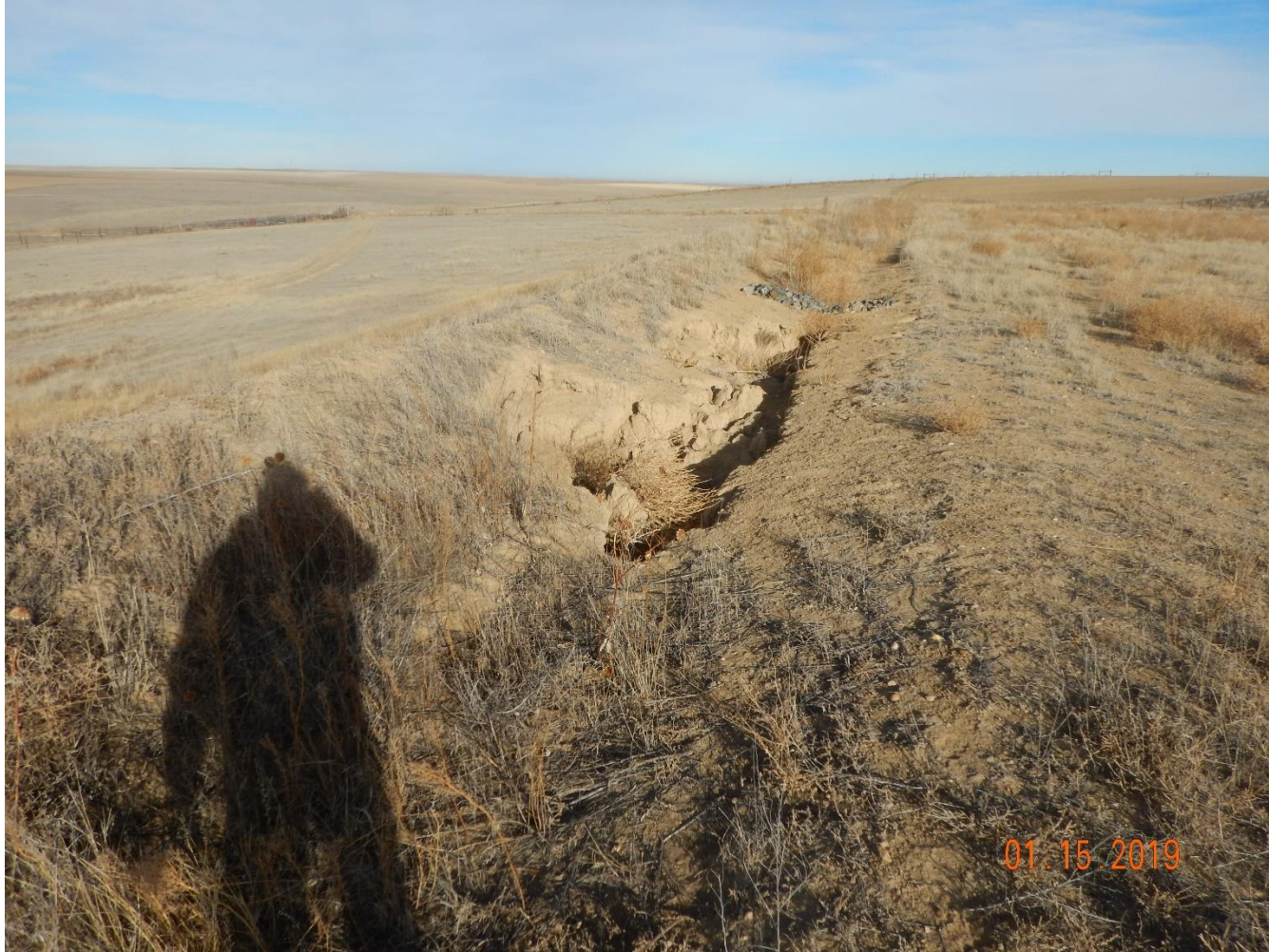
Photo 11: Photo taken from the west end of the location, facing north. Photo shows stormwater degradation within the ditch has not been repaired and stabilized. Stormwater has continued to incise within the ditch and sinkhole appears to have expanded.
