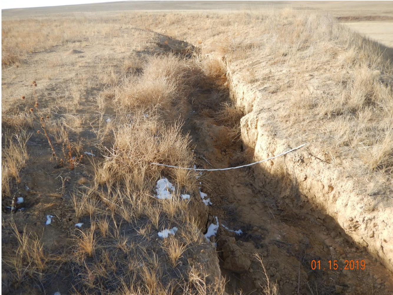
Photo 19: Photo taken from the gully on the northwest end of the pad, facing southwest. Photo shows gully erosion has not been repaired/stabilized. 6 foot measuring stick for reference.
