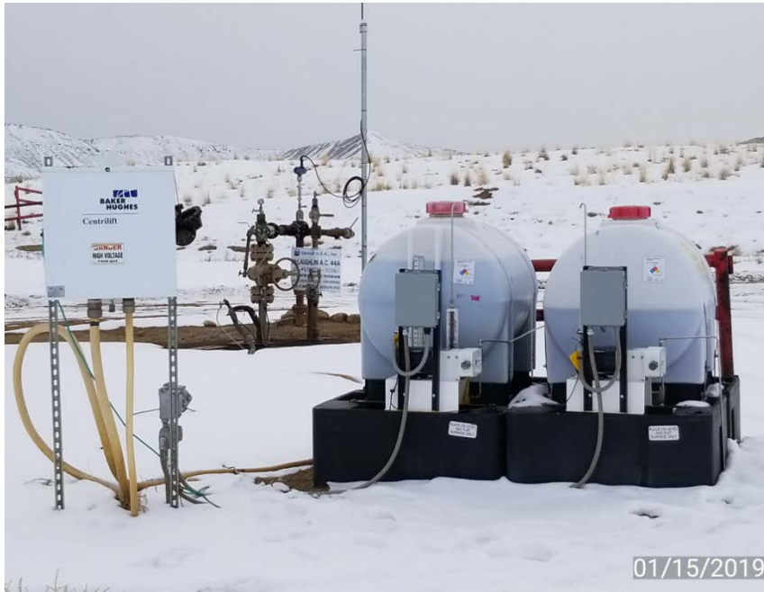
Photo 1. Location looking southwest.
