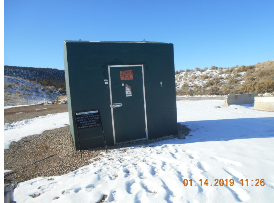
Injection wellhead housing with sign
