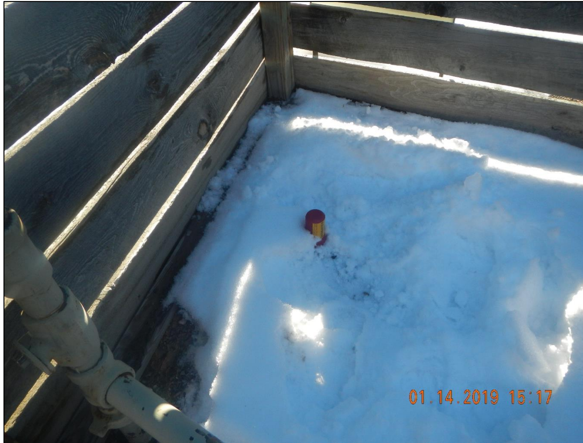
Unused riser capped with a red hammer union cap. Orange "Do not operate" sticker on cap.
