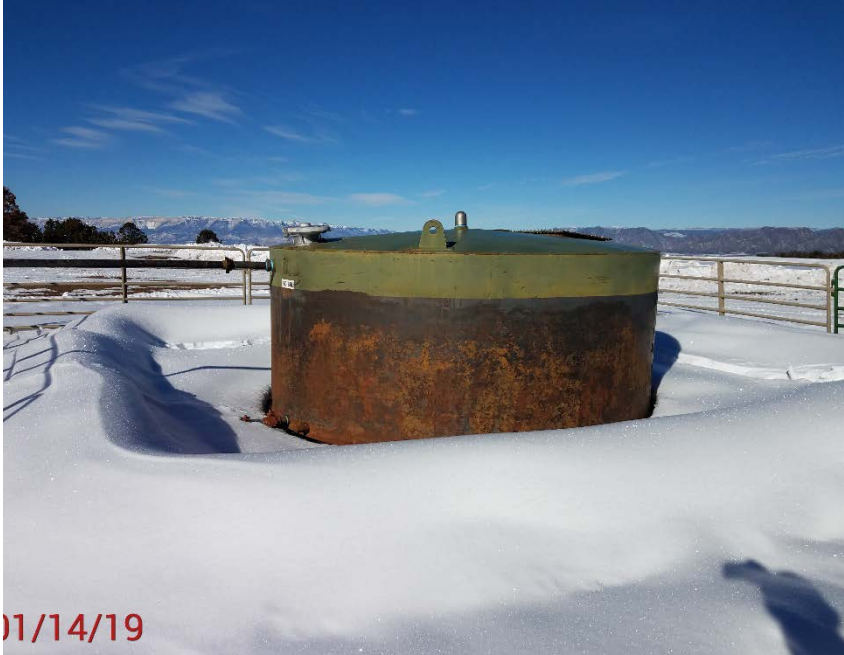
Location Photo #7, Missing labels on tank.
