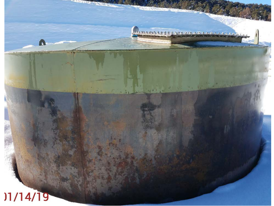
Location Photo #6, Missing labels on tank.
