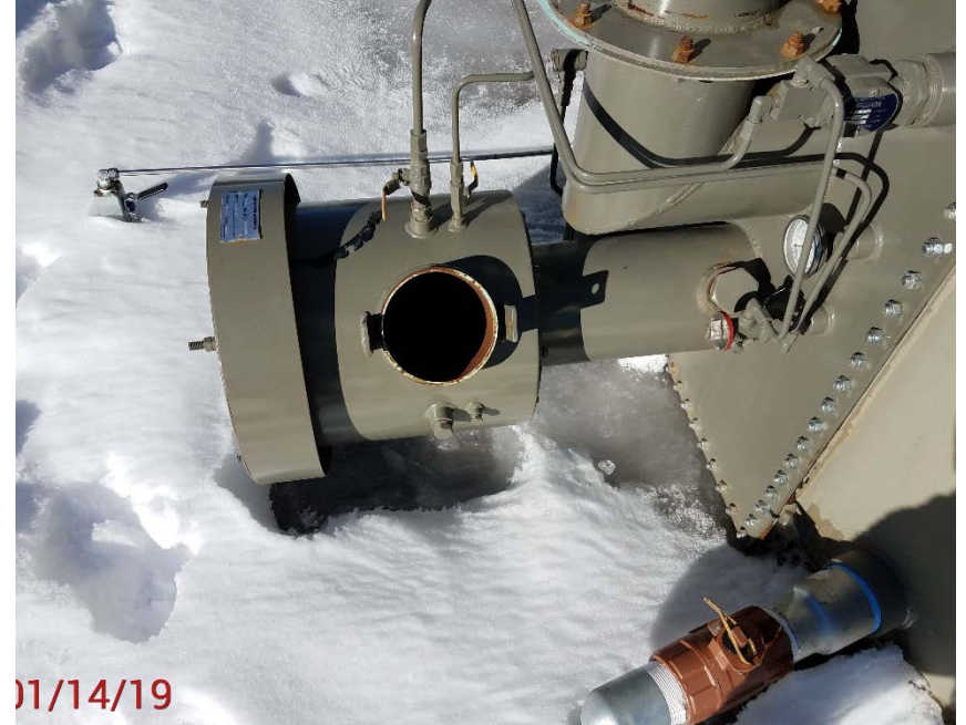
Location Photo #4, missing wildlife screen on tank burner in SE corner.
