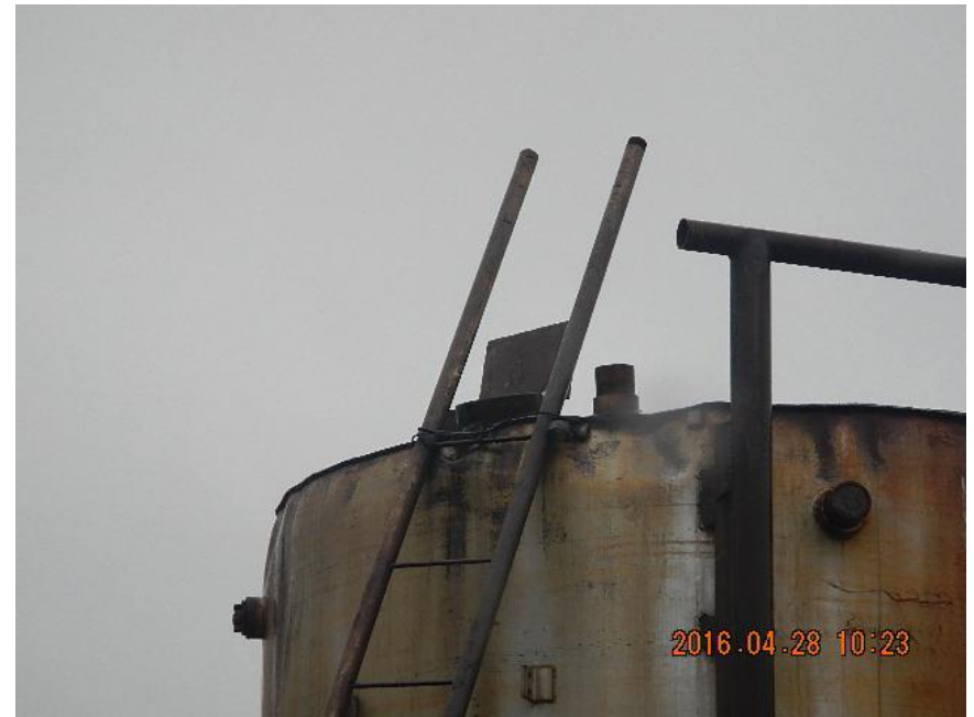
Their hatch open – wellhead valve open as well
