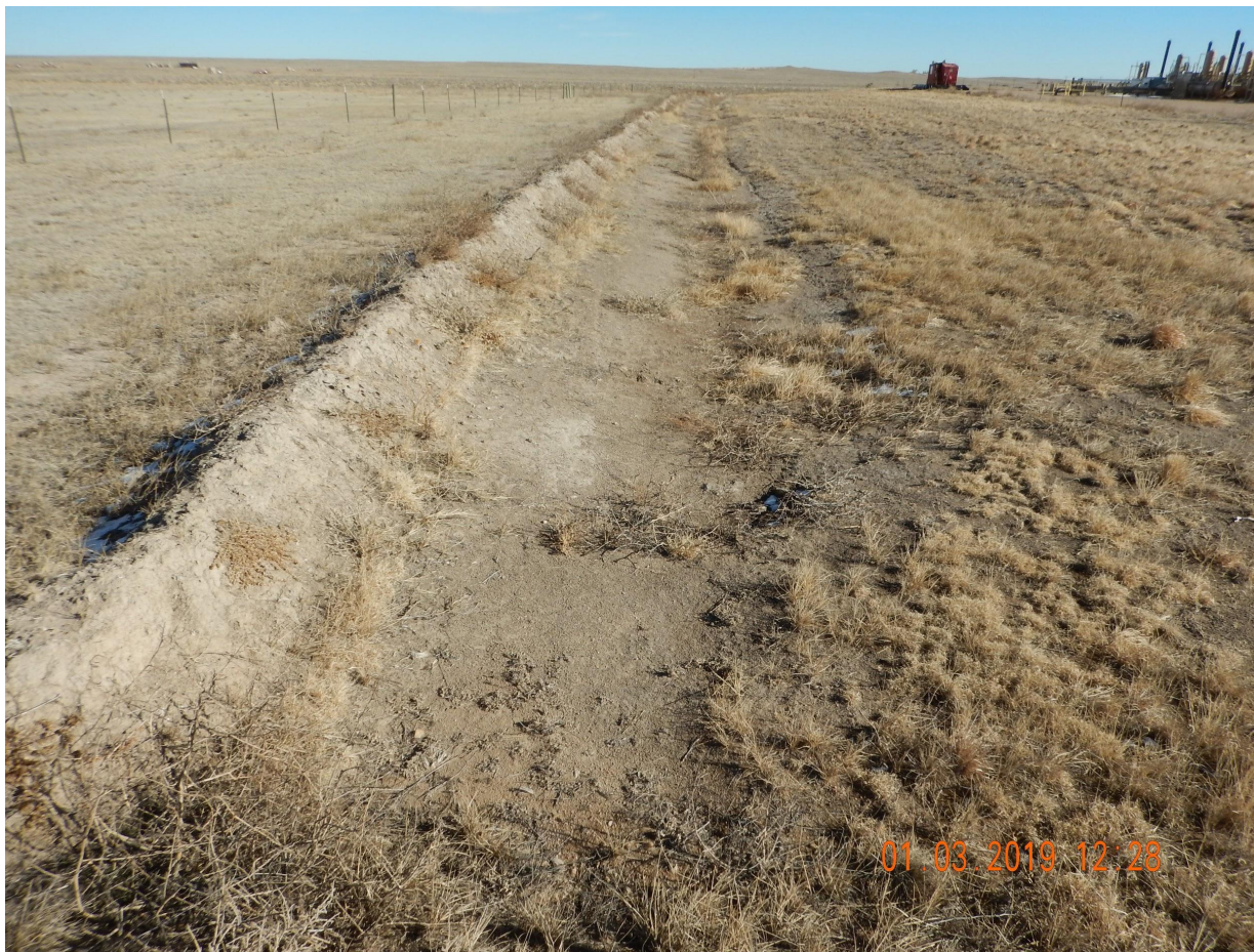
Photo 1. Photo taken from the northwestern location, facing East. Appears the Operator has ditch and berm BMP along the northern location which is directed to a stabilized outlet (sediment trap).
