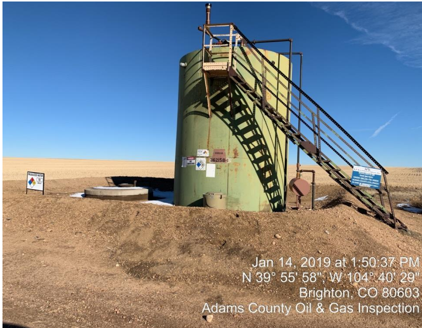
Photo#1 Production Tank and Produced water pit
