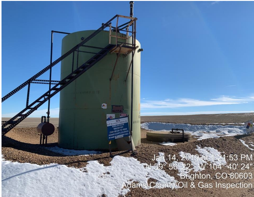
Photo#1 Production Tank and Produced Water Pit
