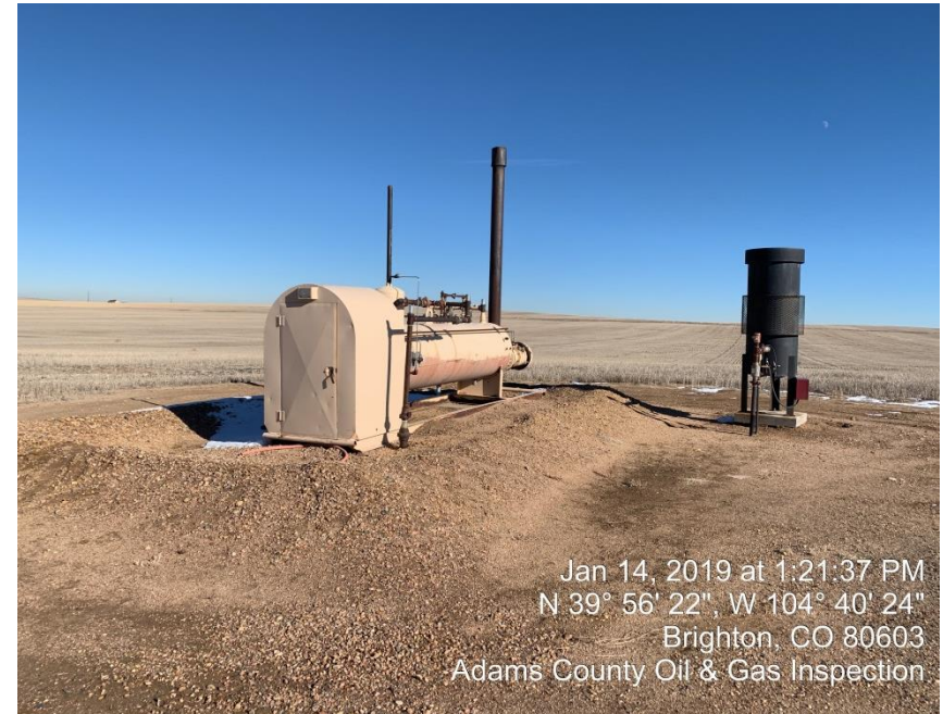
Photo#2 Separator/ECD
