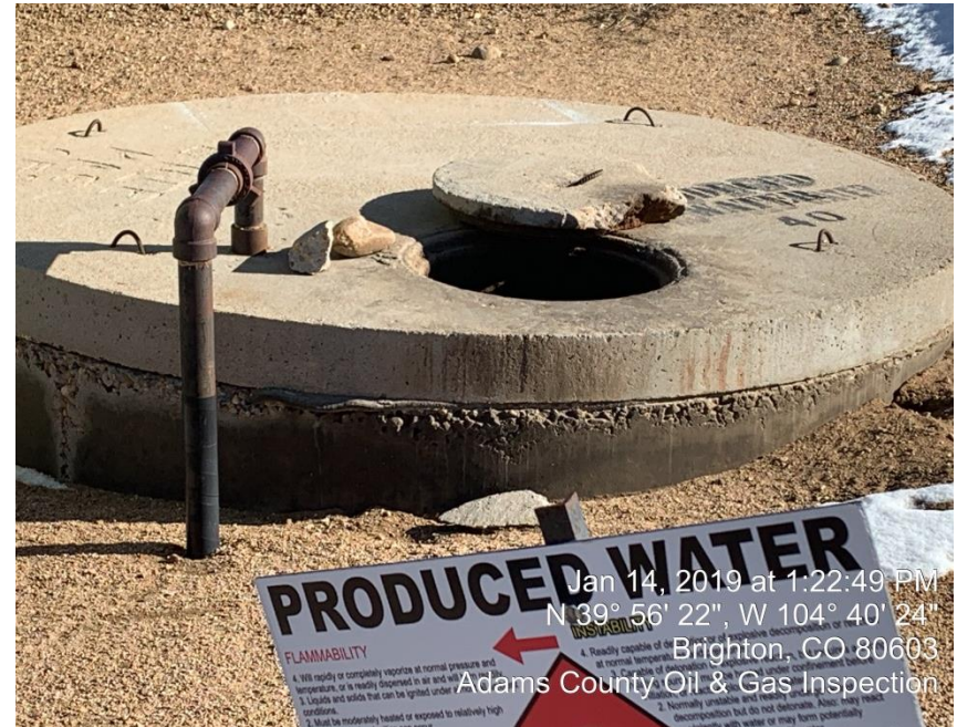
Photo#4 Corrective Action: Cover needs put back on pit
