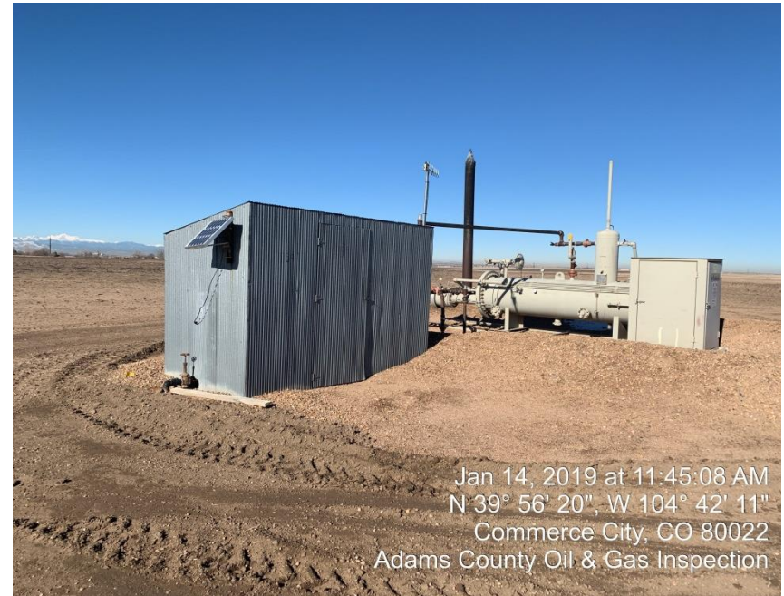
Photo#2 Separator and Gas Meter
