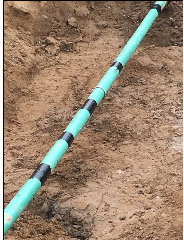
Repairs made to Flowline, Looking west
