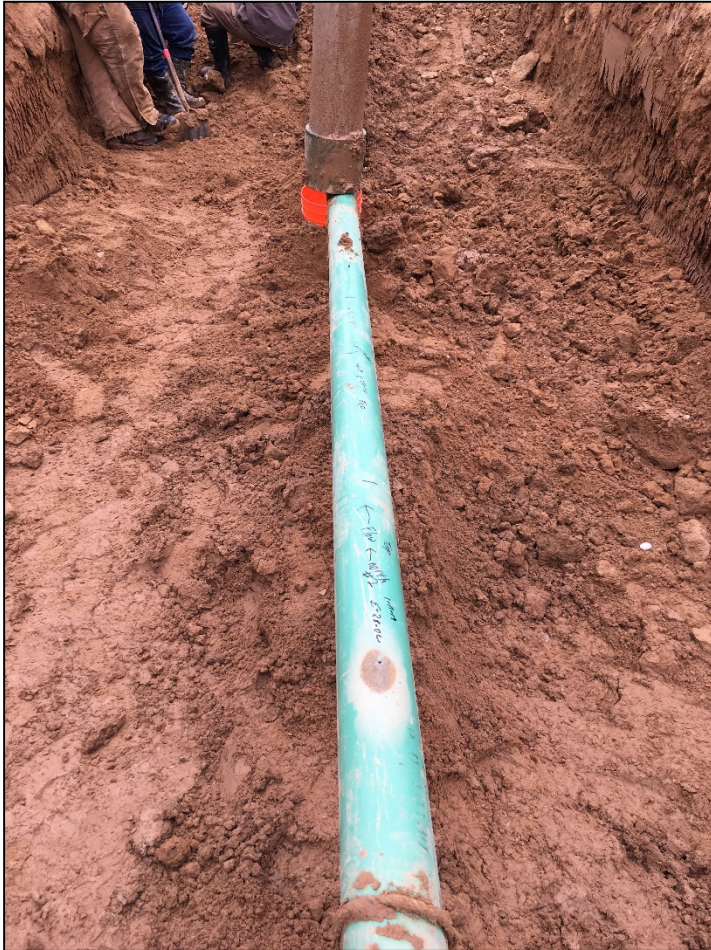
Holes in pipe, 2 nd hole under vac truck hose. Looking east
