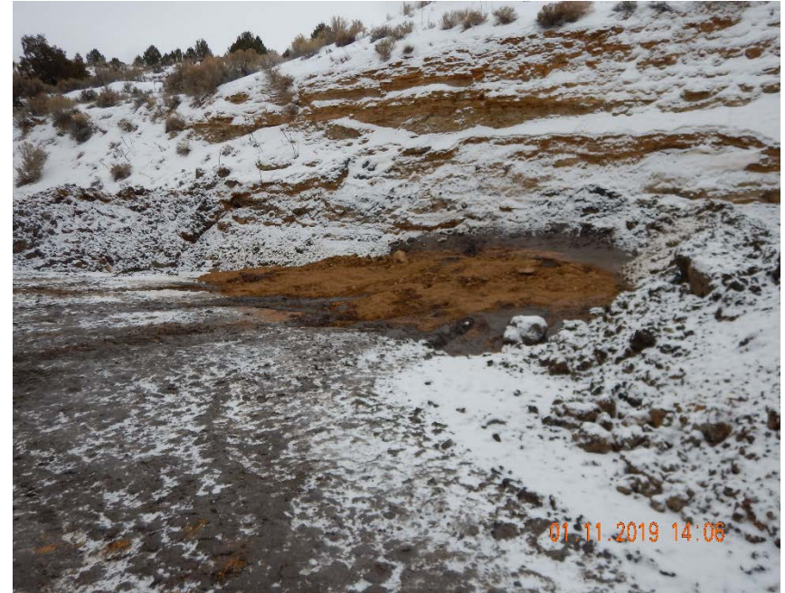
Photo #2 – East bermed drill cuttings storage area. Operator indicated that surface cuttings had been moved from storage area to make room for additional production zone cuttings.
