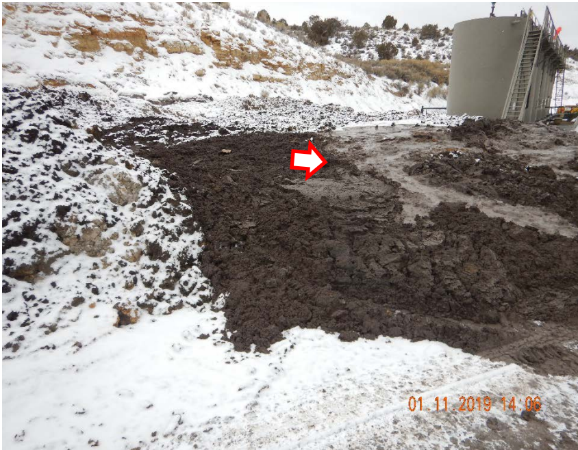
Photo #3 – West bermed drill cuttings area (view from NE) had production zone cuttings on inspection date. Note fluids accumulation on top of cuttings (red arrow).
