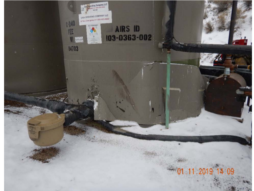
Photo #6 – Western produced water tank had damaged insulation on inspection date.
