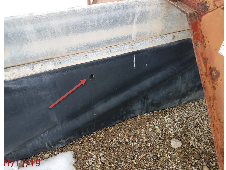
Location Photo #2, Hole in secondary containment liner.
