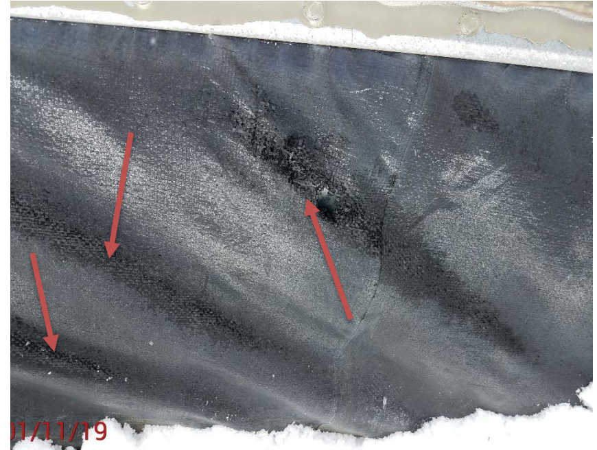
Location Photo #4, Holes in secondary liner, near the stair access point.
